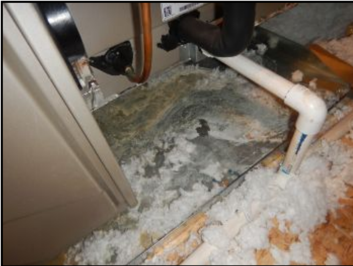
Moisture staining at furnace drip pan.
