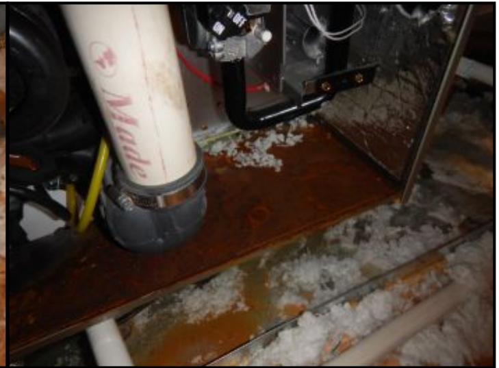
Moisture staining/rust at interior of furnace cabinet.
