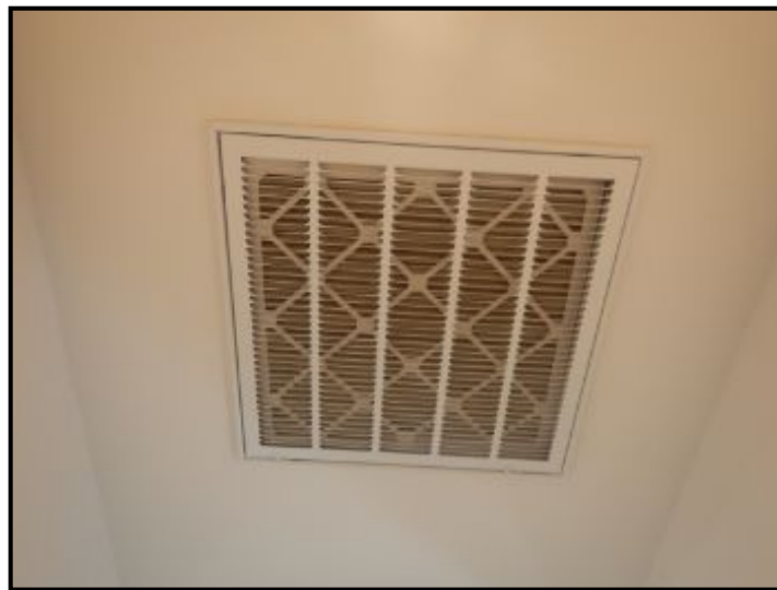
Replace air return filter.
