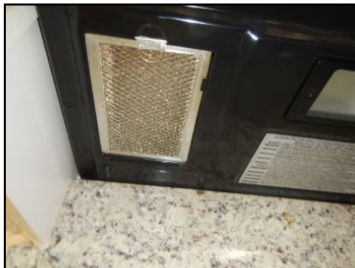
Clean stove top exhaust filters.
