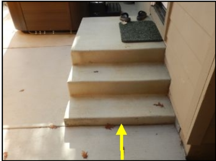
Inconsistent riser height at steps.
