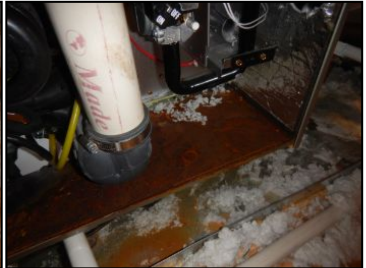
Moisture staining/rust at interior of furnace cabinet.
