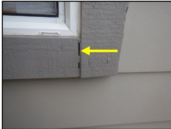
Caulk/seal gaps at exterior trim.
