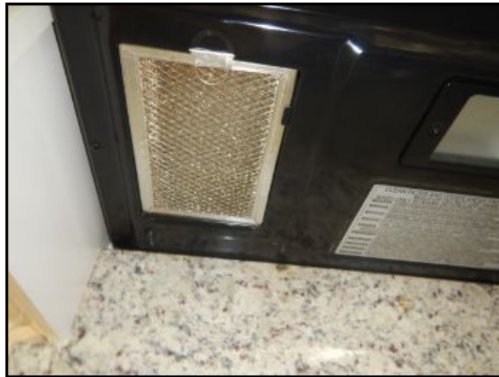
Clean stove top exhaust filters.
