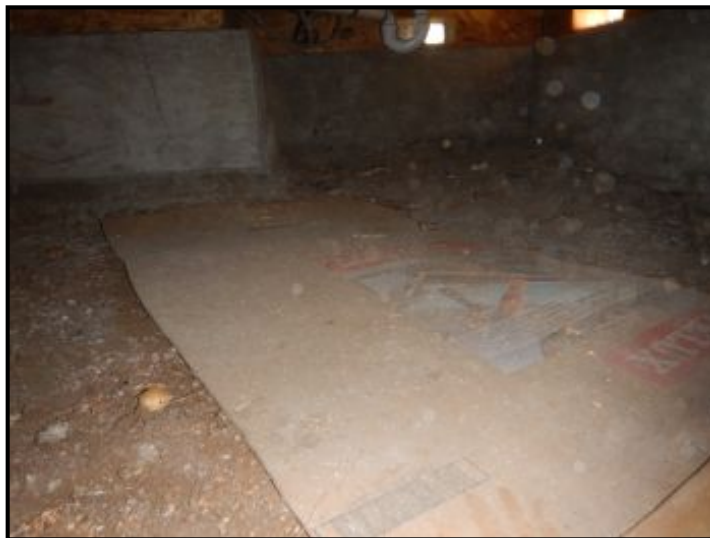
Debris in sub area.
