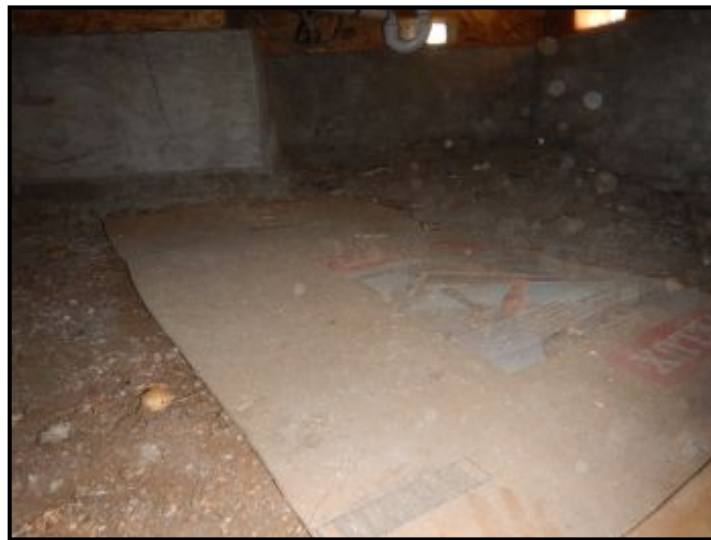
Debris in sub area.
