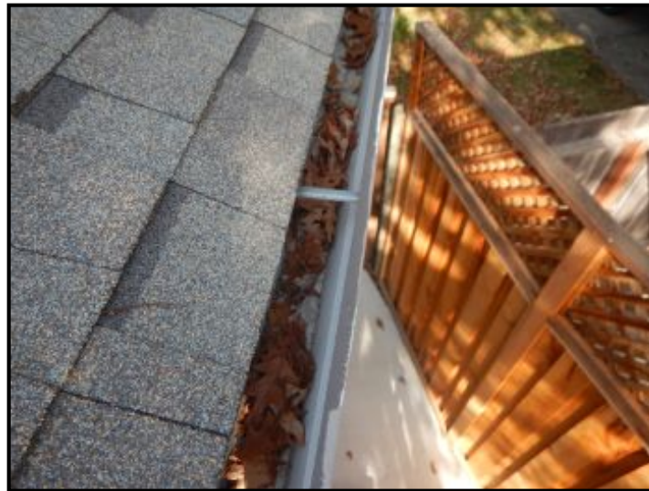
Minor debris in gutters.
