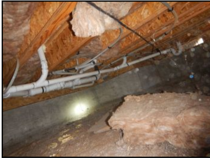
Fallen insulation in sub area.
