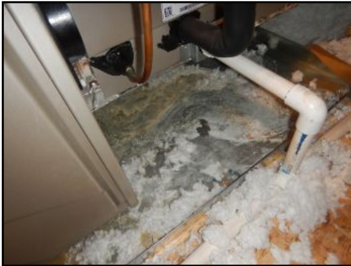
Moisture staining at furnace drip pan.
