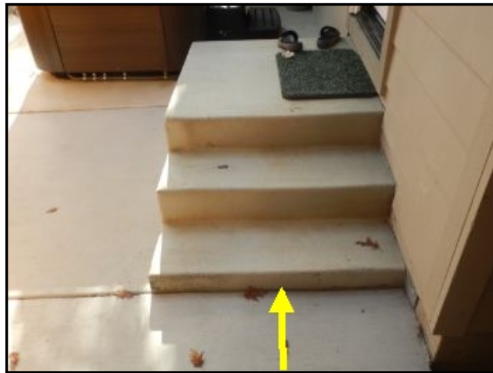
Inconsistent riser height at steps.
