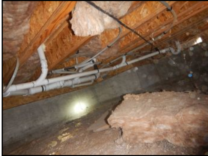
Fallen insulation in sub area.
