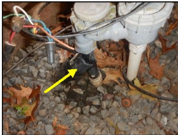
Leaking at exterior irrigation line.
