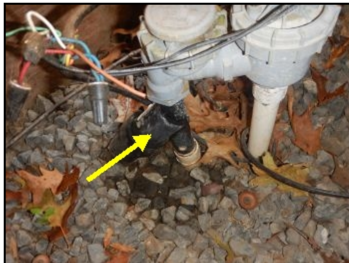
Leaking at exterior irrigation line.
