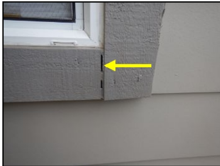
Caulk/seal gaps at exterior trim.
