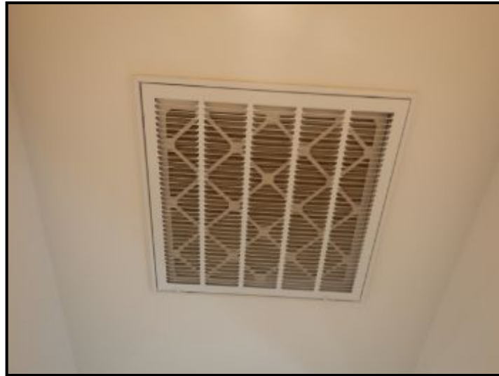
Replace air return filter.
