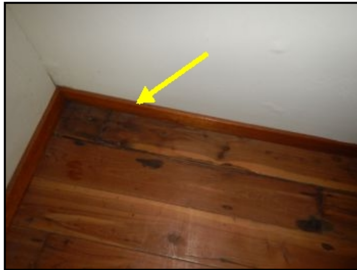
Moisture stains noted in bedroom closet.
