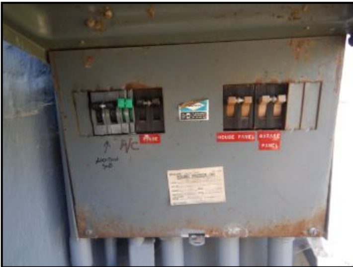
Zinsco panel installed.
