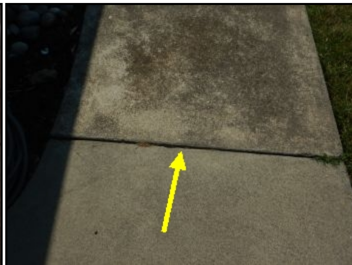
Uneven concrete walkway.
