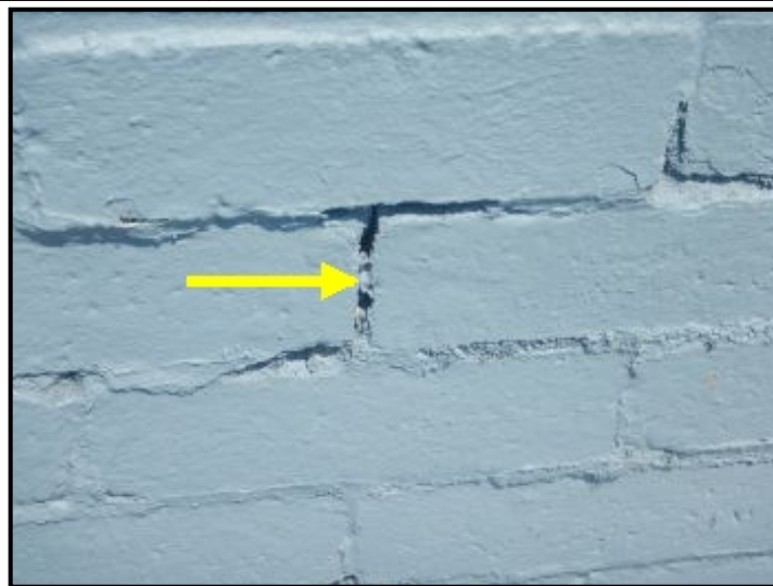
Deterioration of mortar joints at chimney.
