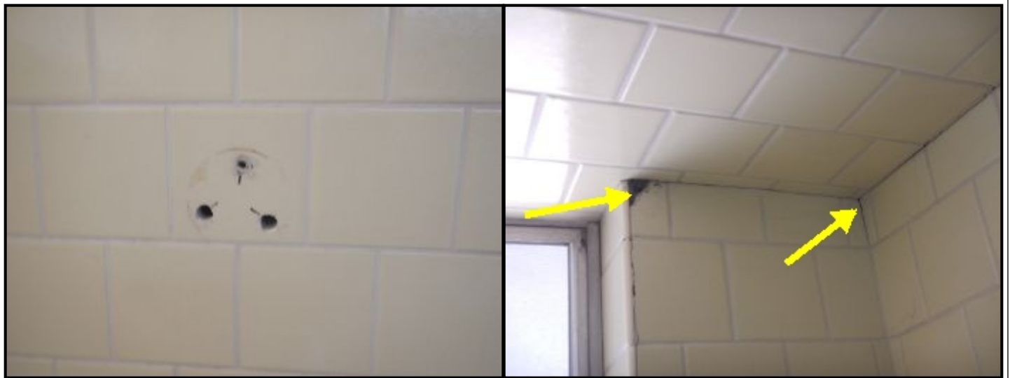
Holes at tile shower wall.
