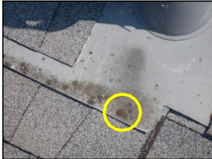
Seal exposed fasteners at roof top flashings.
