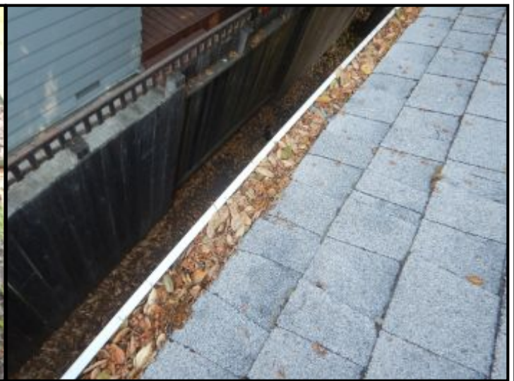
Debris build up in gutters.
