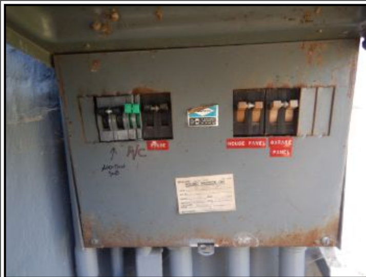
Zinsco panel installed.
