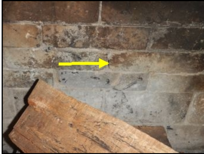
Deterioration of mortar joints at interior of fireplace.
