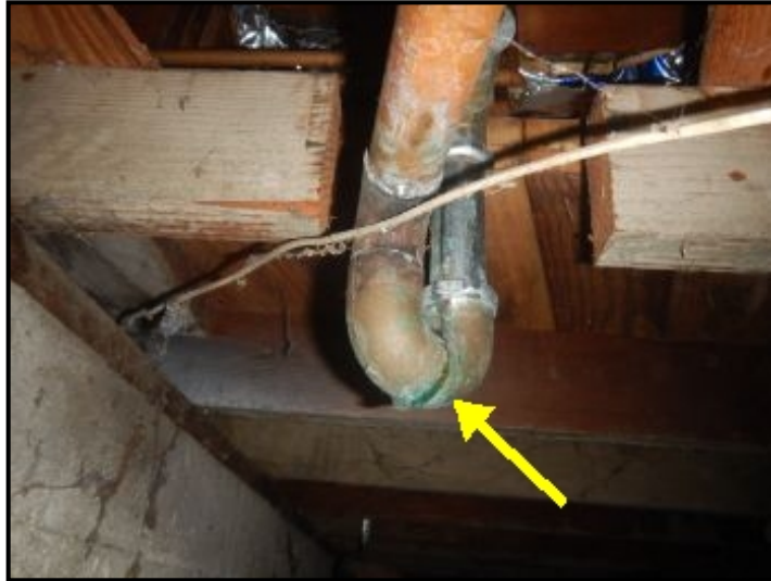
Leaking at shower drain line.
