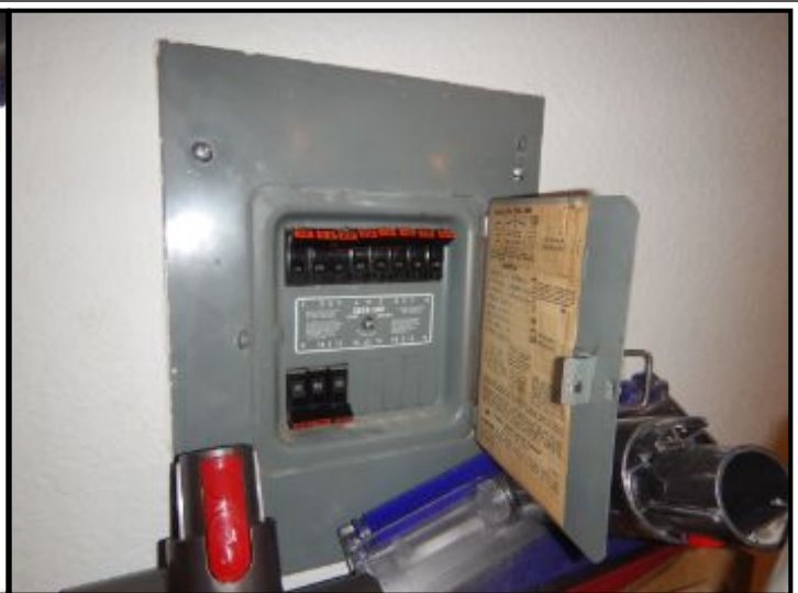
Federal Pacific panel installed.
