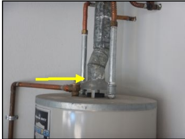
No screws installed at flue/flue hood.
