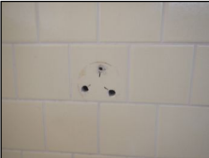
Holes at tile shower wall.
