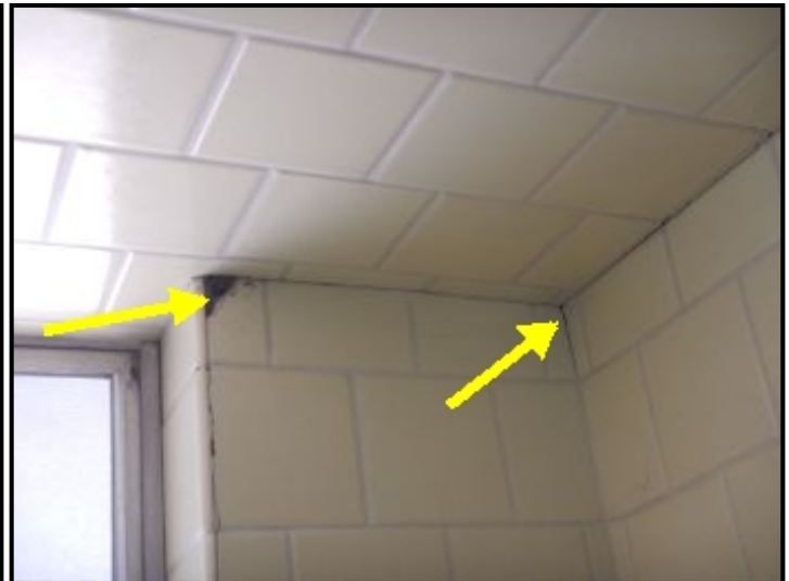
Grout voids/damaged tiles at shower wall.
