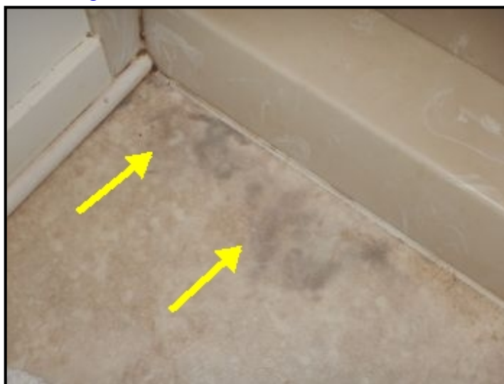
Suspect moisture intrusion under bathroom floor cover.
