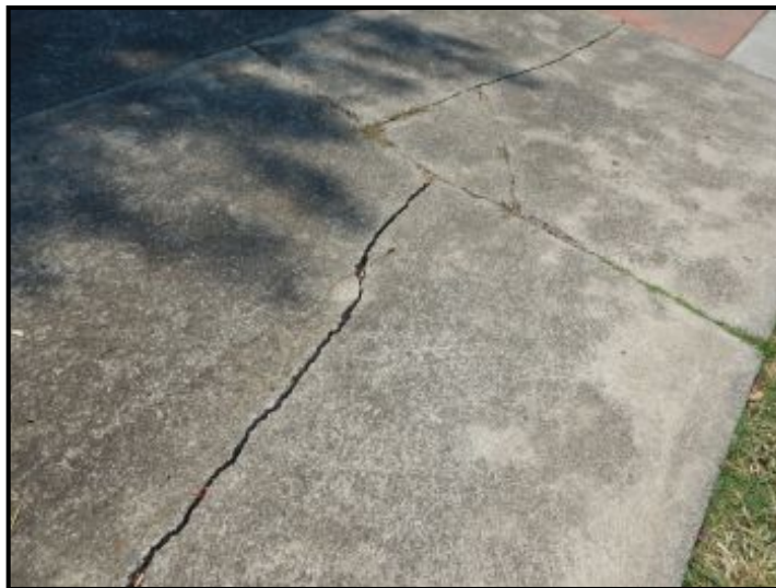
Cracking concrete at driveway.
