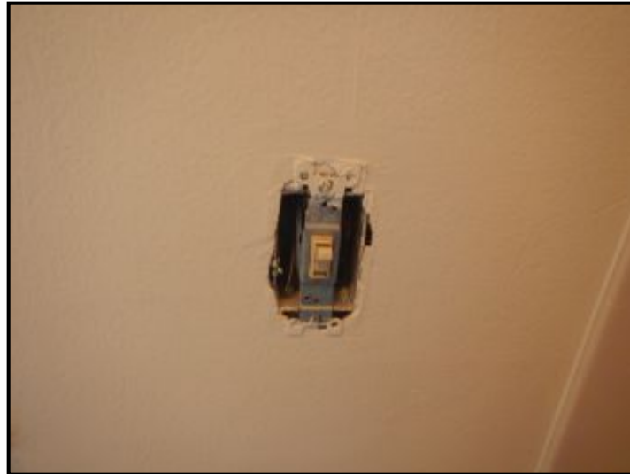
Missing cover plates at various areas.
