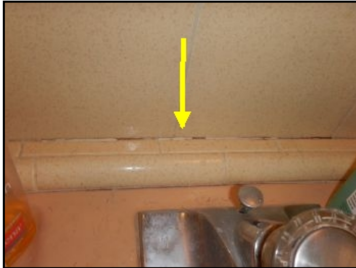
Grout voids at bathroom counter top.
