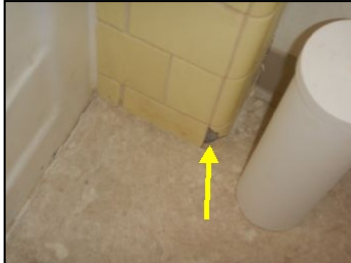
Damaged tile at shower wall.
