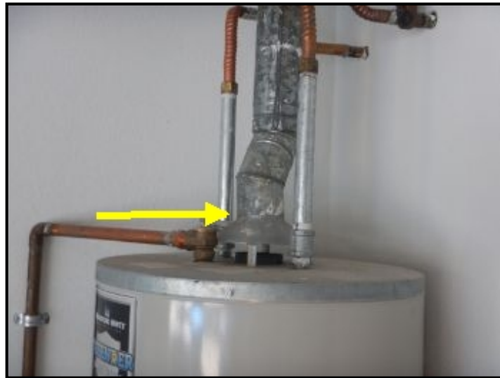
No screws installed at flue/flue hood.
