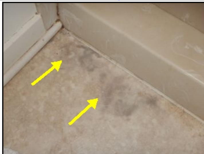
Suspect moisture intrusion under bathroom floor cover.
