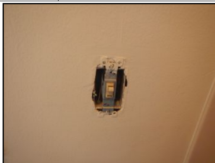
Missing cover plates at various areas.
