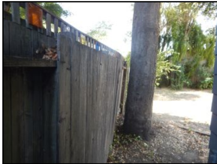
Leaning fence at left side of home.
