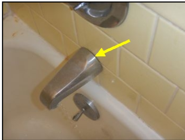
Caulk and seal around tub spout.
