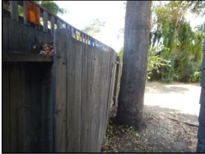
Leaning fence at left side of home.
