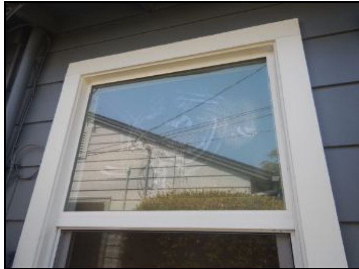
Lost seal at window.
