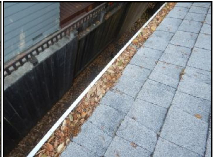
Debris build up in gutters.
