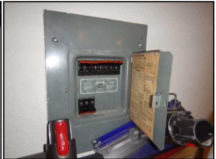
Federal Pacific panel installed.
