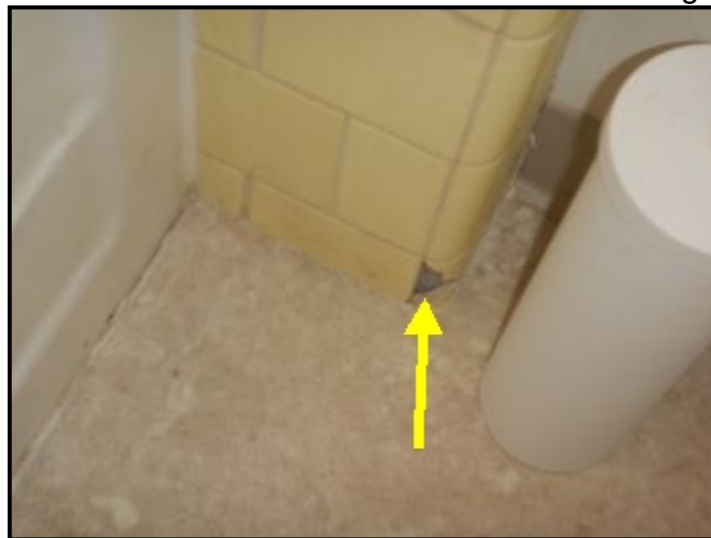
Damaged tile at shower wall.
