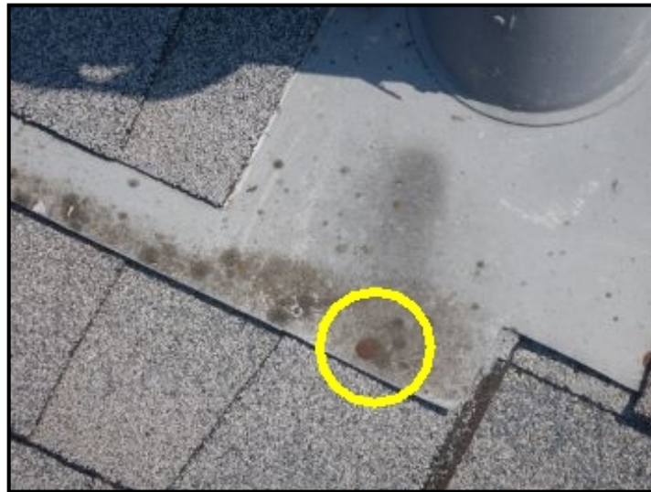
Seal exposed fasteners at roof top flashings.
