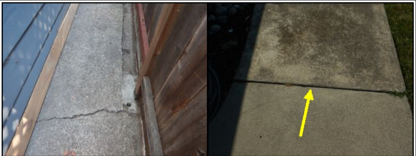
Cracking at concrete walkways.
