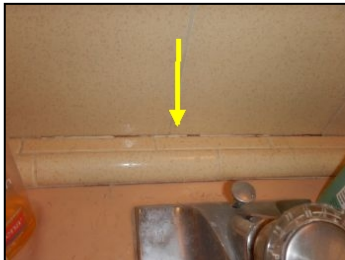
Grout voids at bathroom counter top.
