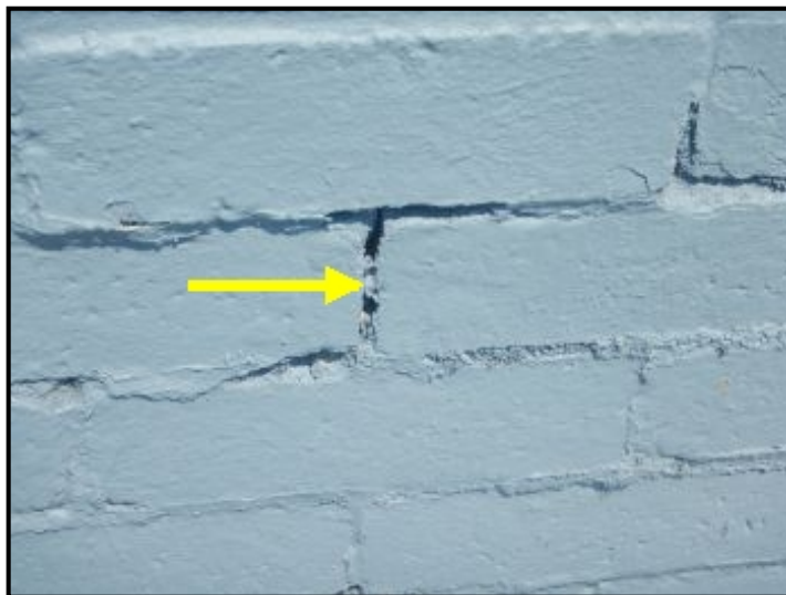
Deterioration of mortar joints at chimney.
