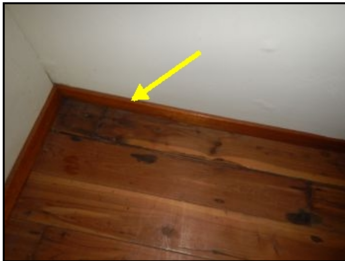
Moisture stains noted in bedroom closet.
