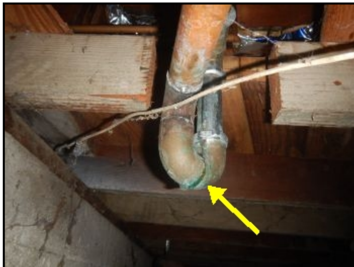
Leaking at shower drain line.
