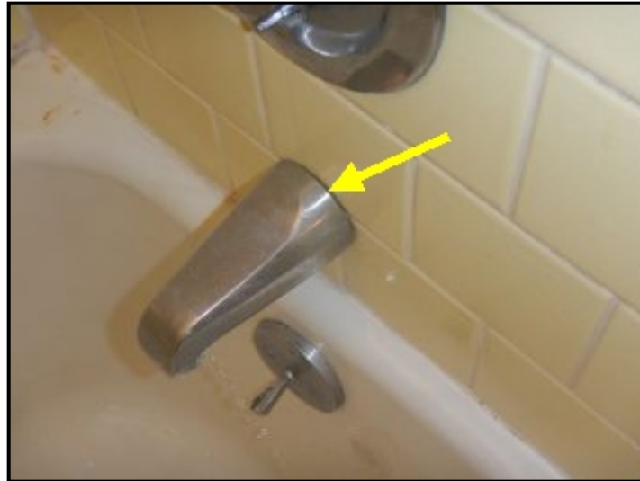
Caulk and seal around tub spout.
