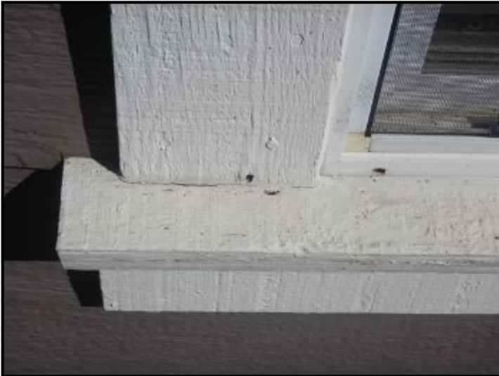
Window trim damage at side of garage.
