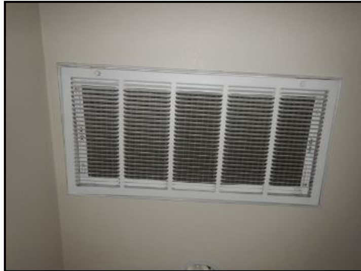
Replace air return filter.
