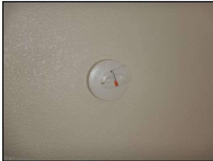
Missing battery at smoke detector.
