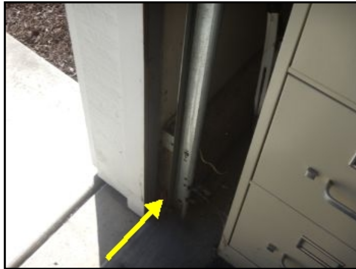
Loose track at garage door.
