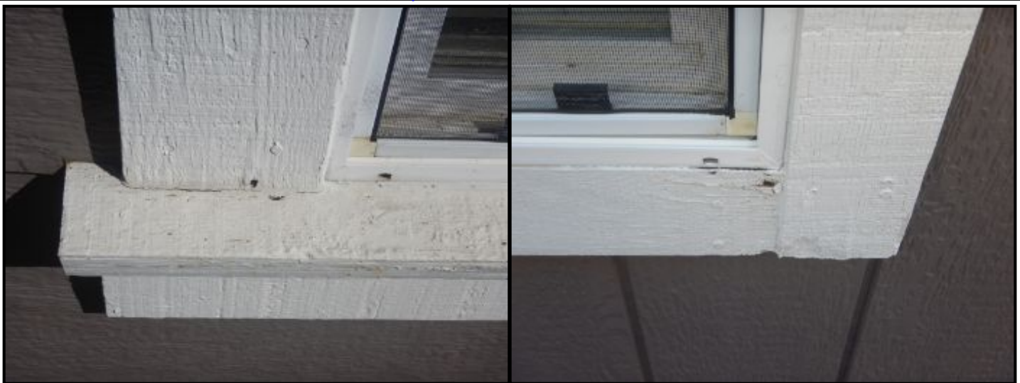
Window trim damage at side of garage.
