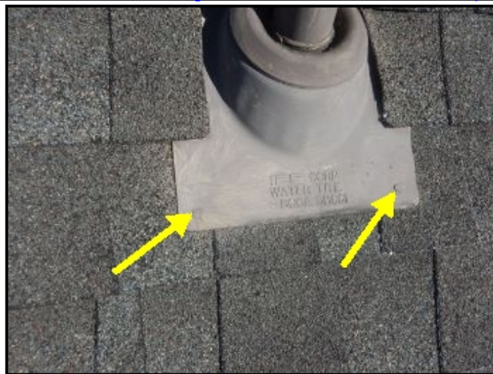
Seal exposed fasteners at flashings.
