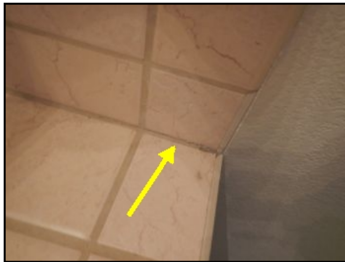
Cracking grout at bathroom counter top.
