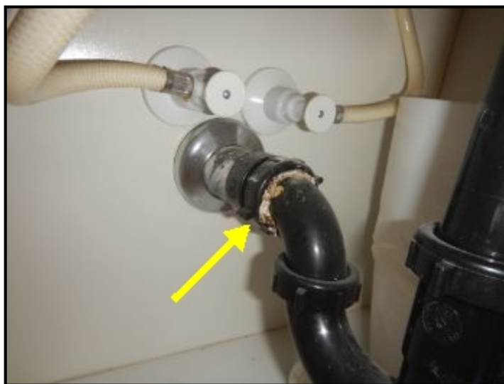
Leaking at bathroom sink drain line.
