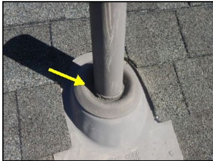
Collapsed storm collar at plumbing vents.
