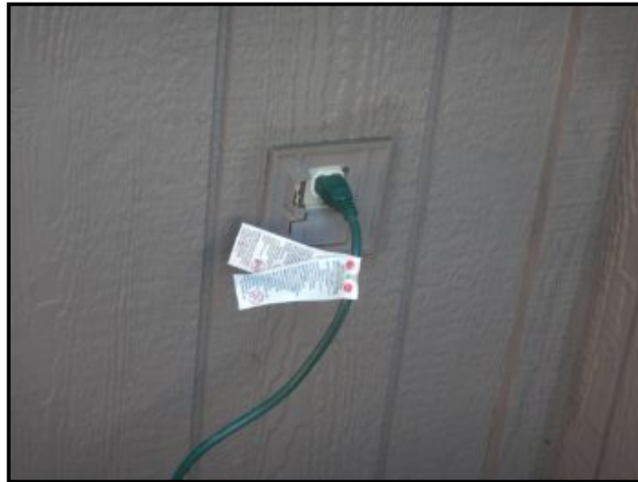
Damaged cover at rear patio.
