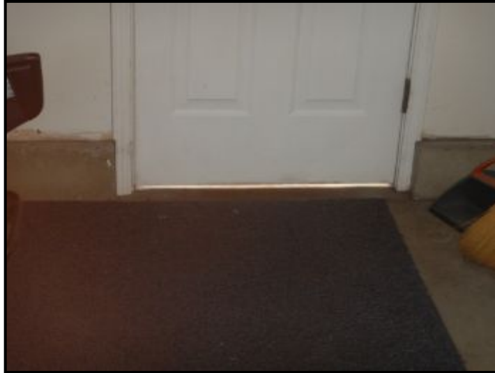
Gaps under side garage door.
