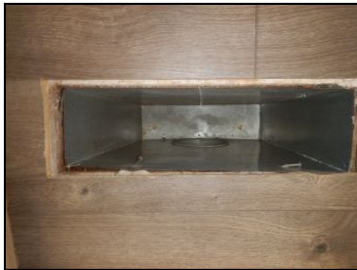
Recommend taping gaps around heat registers.
