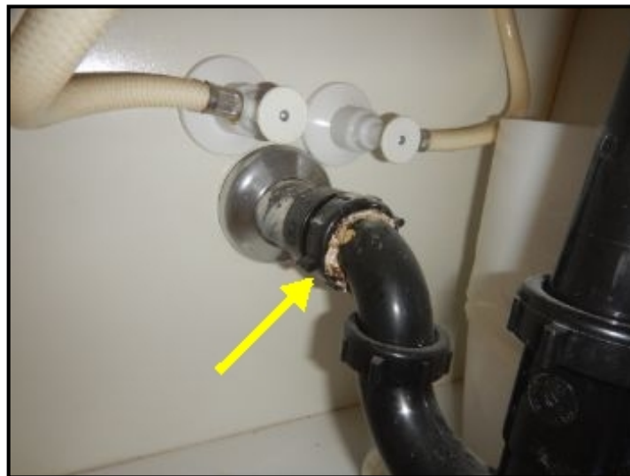
Leaking at bathroom sink drain line.
