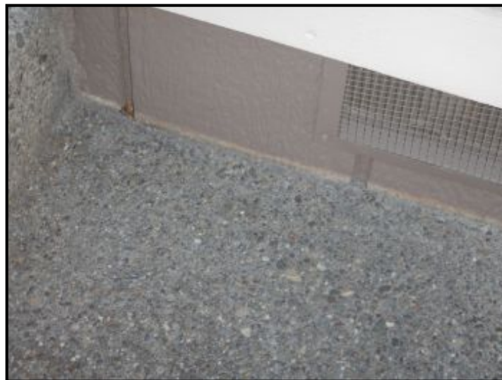
Siding installed behind concrete steps.
