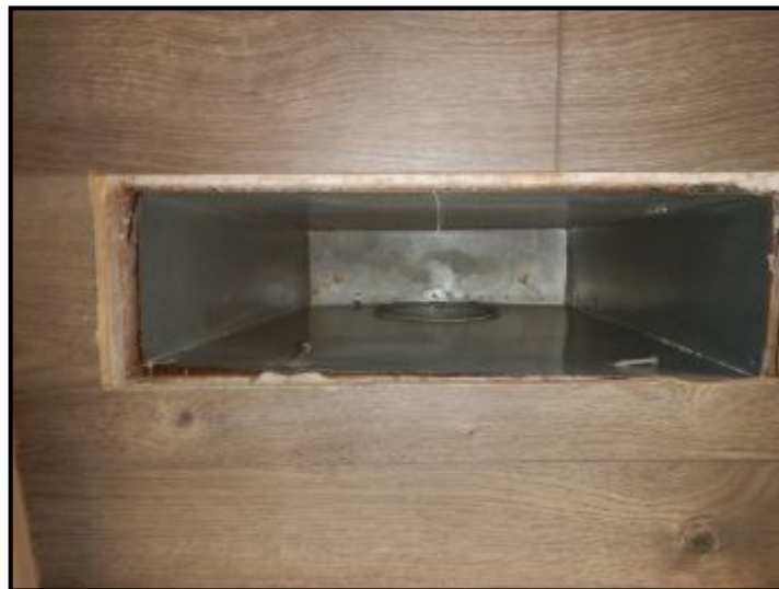
Recommend taping gaps around heat registers.
