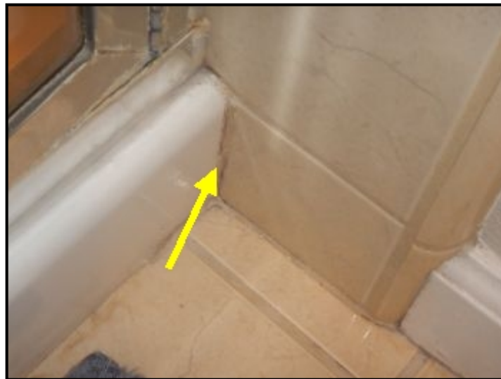
Grout voids at exterior of shower.
