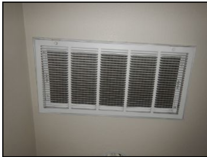
Replace air return filter.
