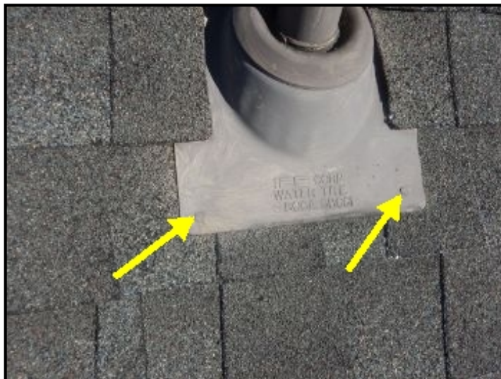
Seal exposed fasteners at flashings.
