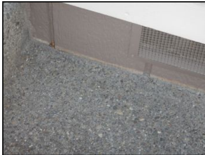
Siding installed behind concrete steps.
