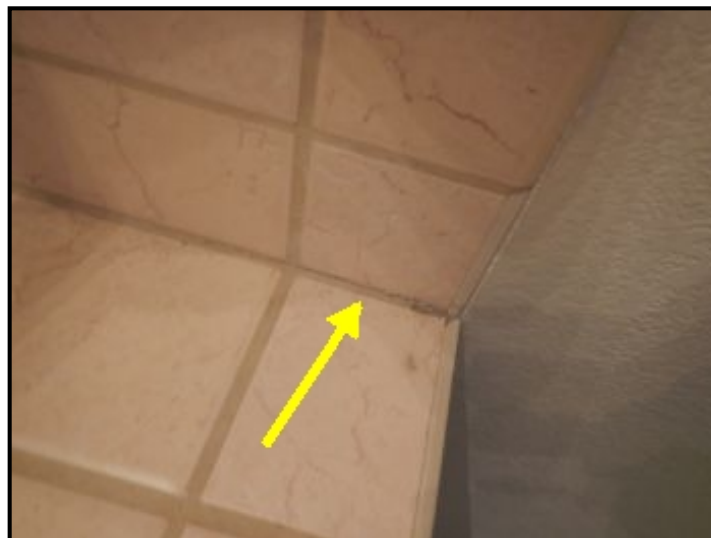
Cracking grout at bathroom counter top.
