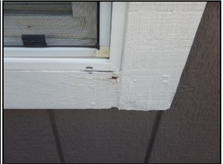
Window trim damage at side of home.
