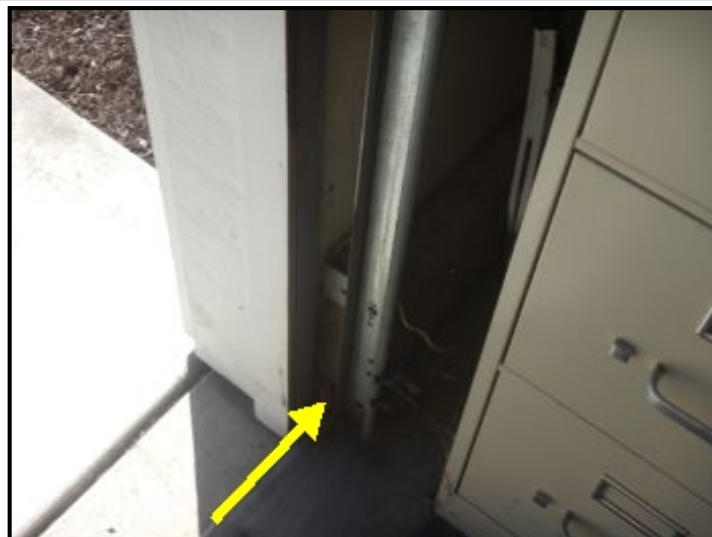
Loose track at garage door.
