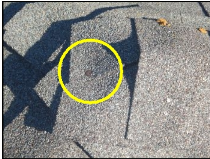
Seal fasteners at ridge shingles.
