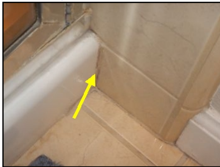
Grout voids at exterior of shower.
