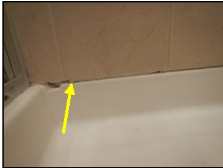
Caulking touch ups needed.
