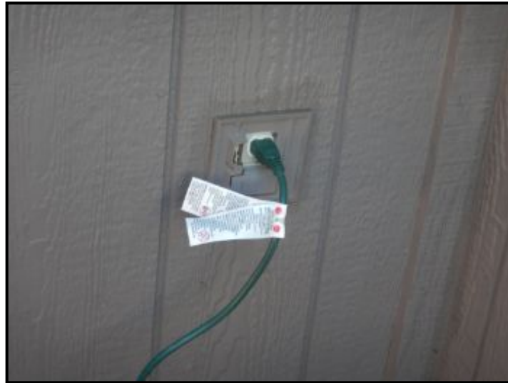
Damaged cover at rear patio.
