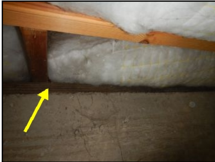
Insulation blocking vents.
