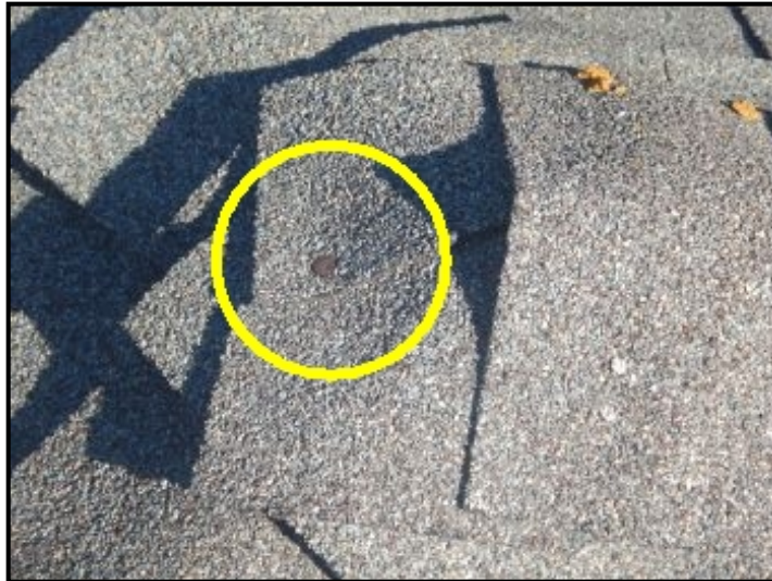
Seal fasteners at ridge shingles.
