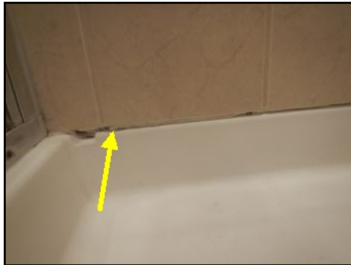
Caulking touch ups needed.
