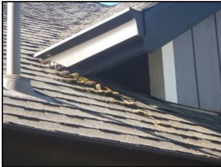
Moss growth on roof top.
