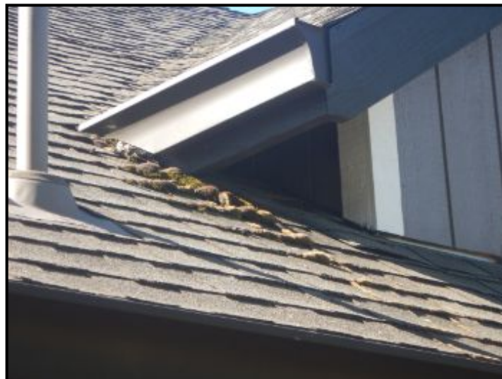
Moss growth on roof top.
