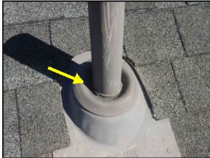
Collapsed storm collar at plumbing vents.
