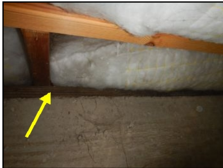
Insulation blocking vents.
