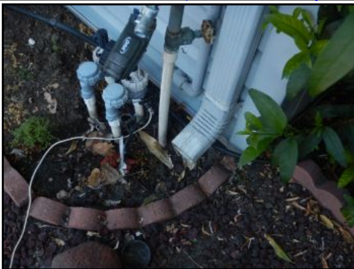
Gutters draining at foundation wall.
