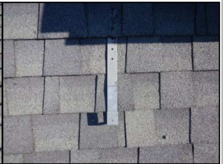
Exposed fasteners at brackets.
