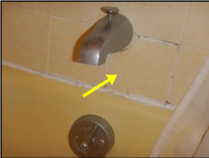
Cracked tiles at bathroom shower.
