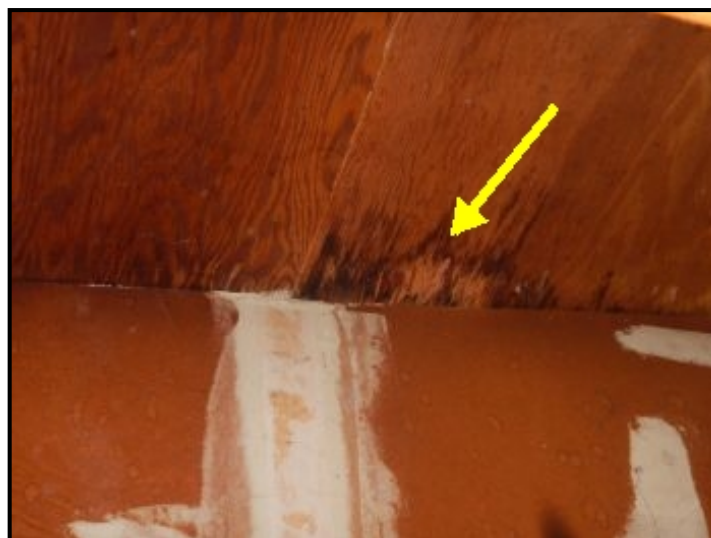
Moisture staining at garage ceiling.
