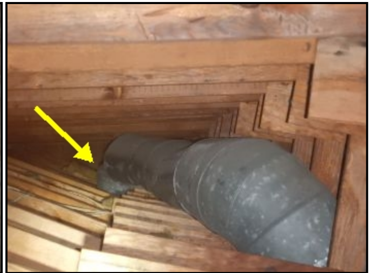
Disconnected air return in attic.
