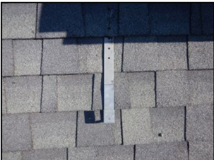
Exposed fasteners at brackets.
