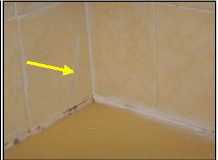
Cracked tiles at bathroom shower.
