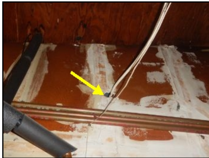
Seal all holes at firewall.
