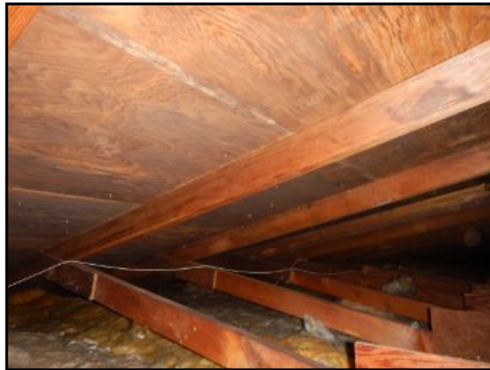
Discoloration to framing in attic.
