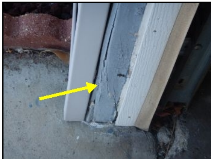
Split trim at garage door.
