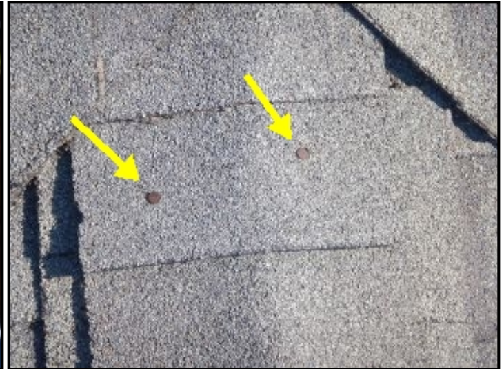
Exposed ridge fasteners.
