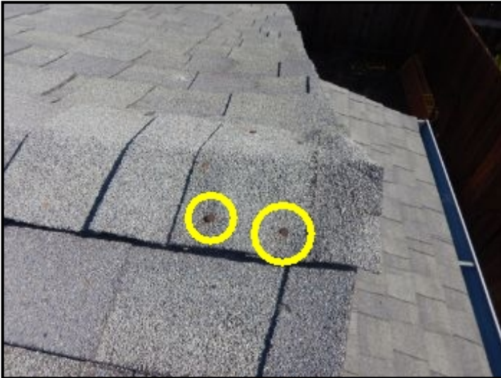
Exposed fasteners at ridge shingles.
