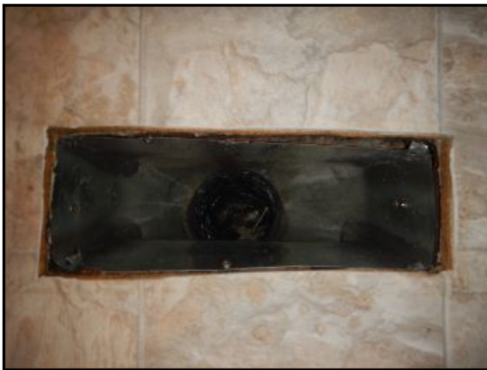
Seal gaps around the floor heat registers.
