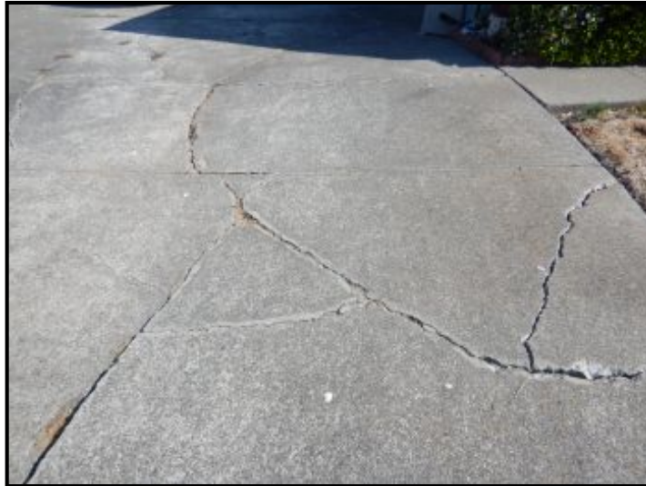
Excessive cracking to driveway.
