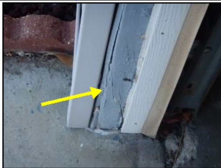
Split trim at garage door.
