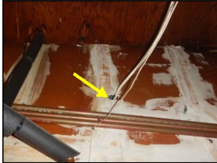
Seal all holes at firewall.
