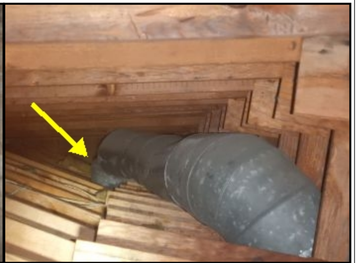
Disconnected air return in attic.
