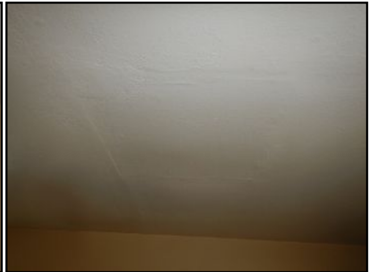
Patch marks at living room ceiling.
