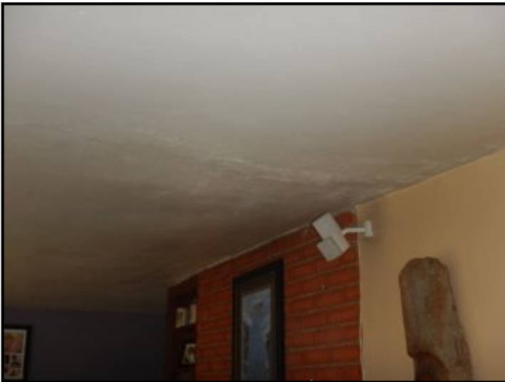
Sagging ceiling in living room.
