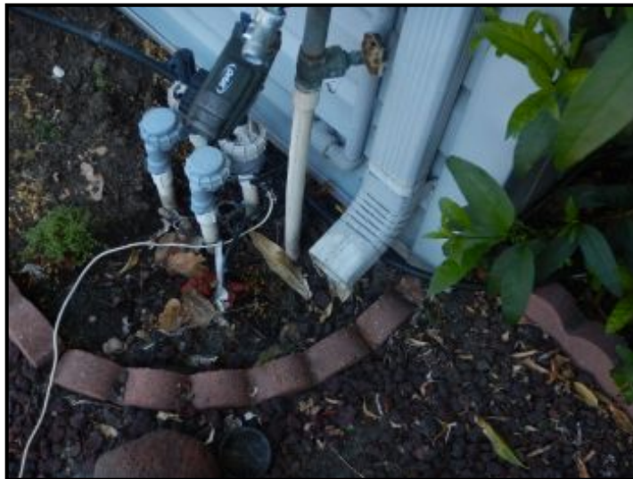
Gutters draining at foundation wall.
