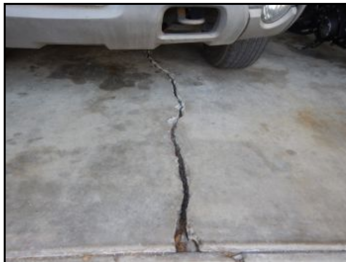
Cracking at garage floor.
