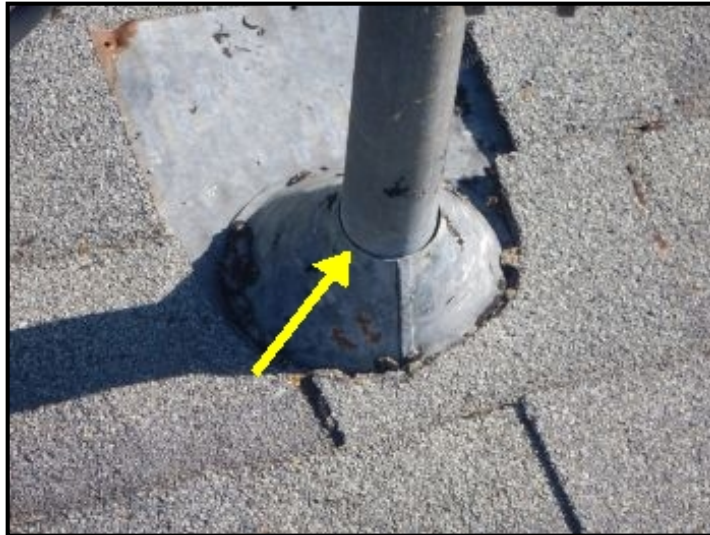
Seal around main electrical drop.
