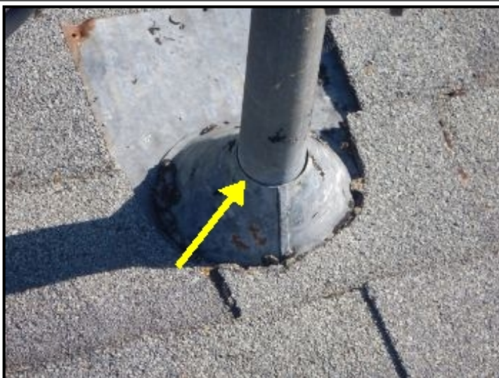
Seal around main electrical drop.
