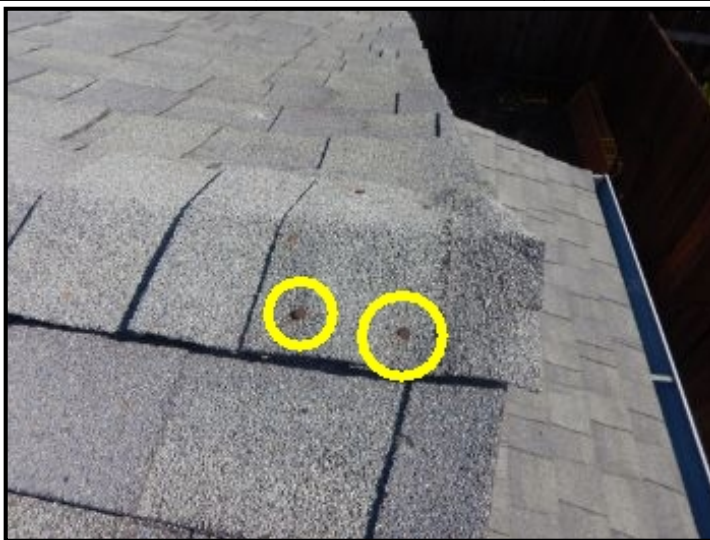
Exposed fasteners at ridge shingles.
