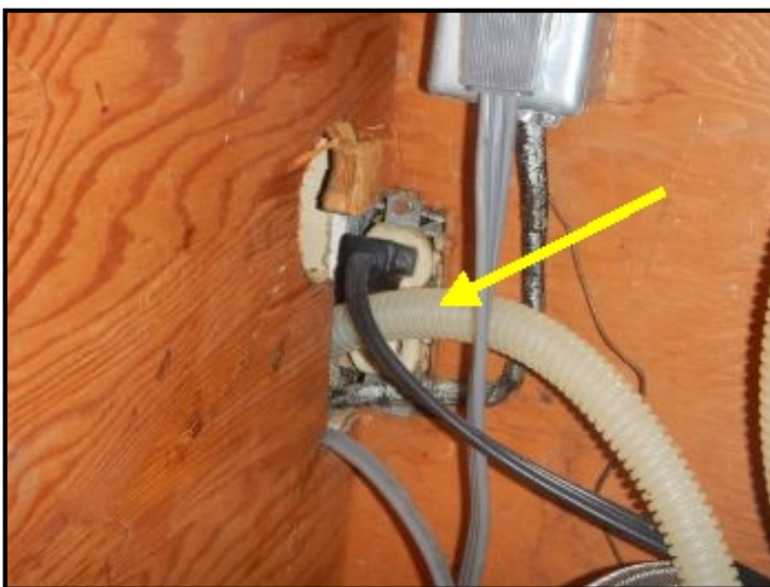
Missing cover plate under the kitchen sink.
