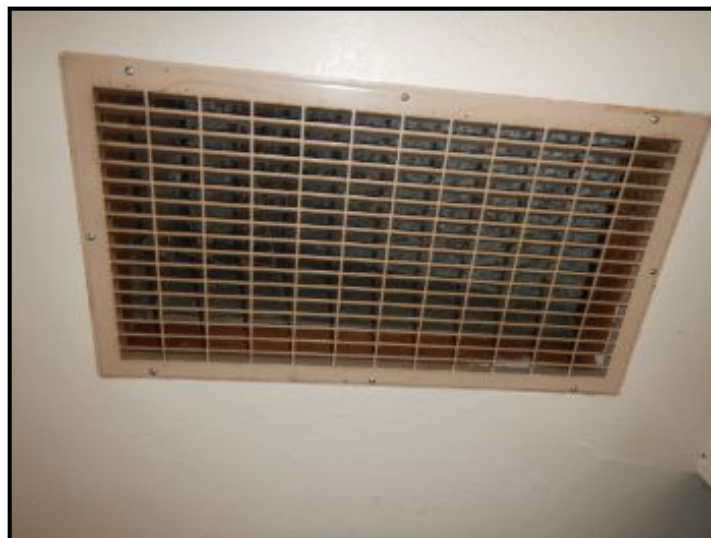
No filter installed at air return.
