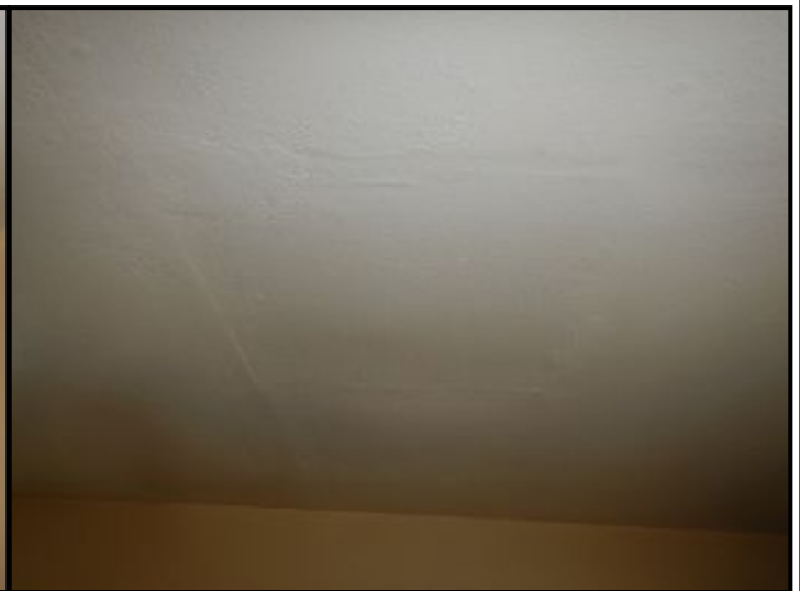
Patch marks at living room ceiling.
