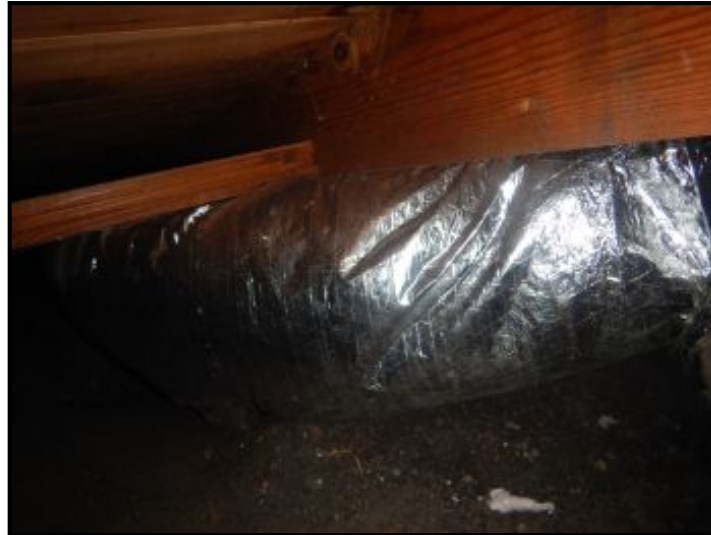
Heating ducts sitting on ground in sub area.
