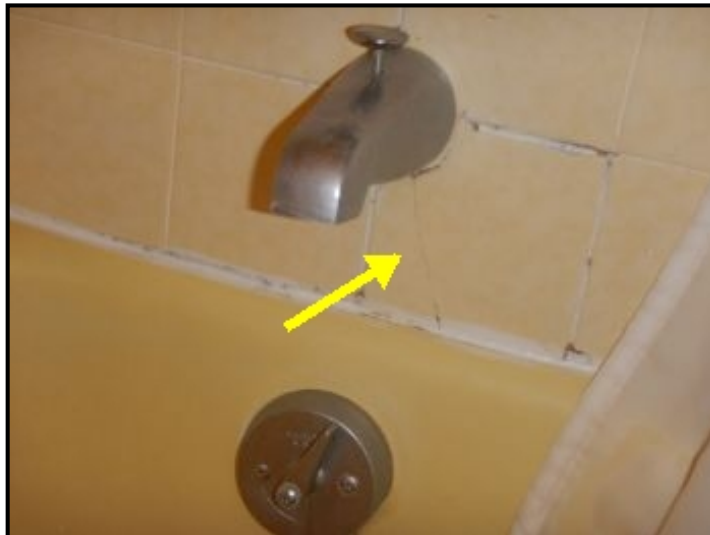
Cracked tiles at bathroom shower.
