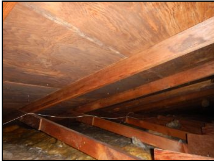
Discoloration to framing in attic.
