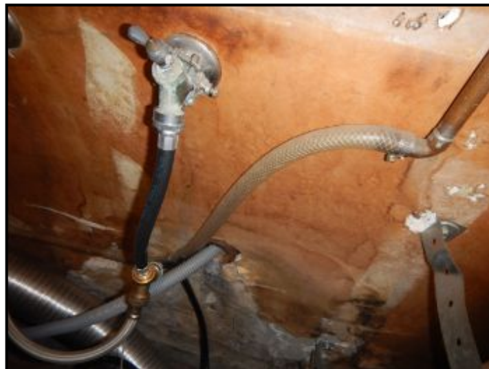
Indications of past leaking washing machine drain line.
