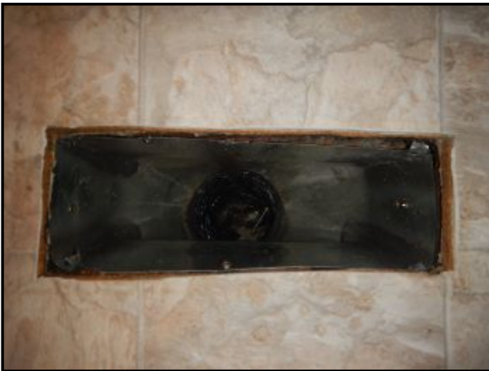
Seal gaps around the floor heat registers.
