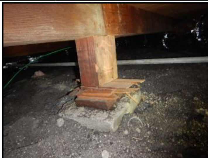
Shims used at concrete piers.
