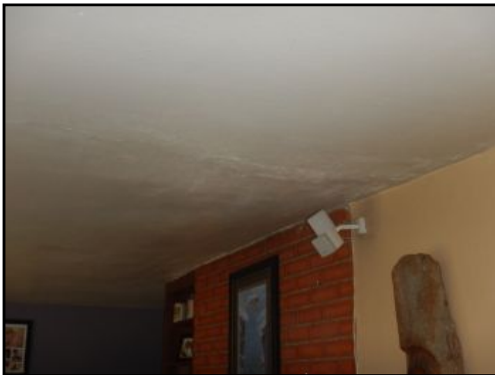
Sagging ceiling in living room.
