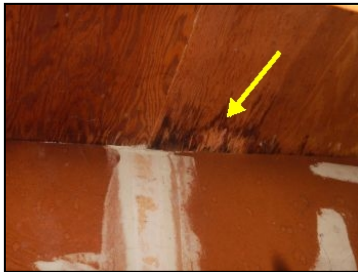
Moisture staining at garage ceiling.
