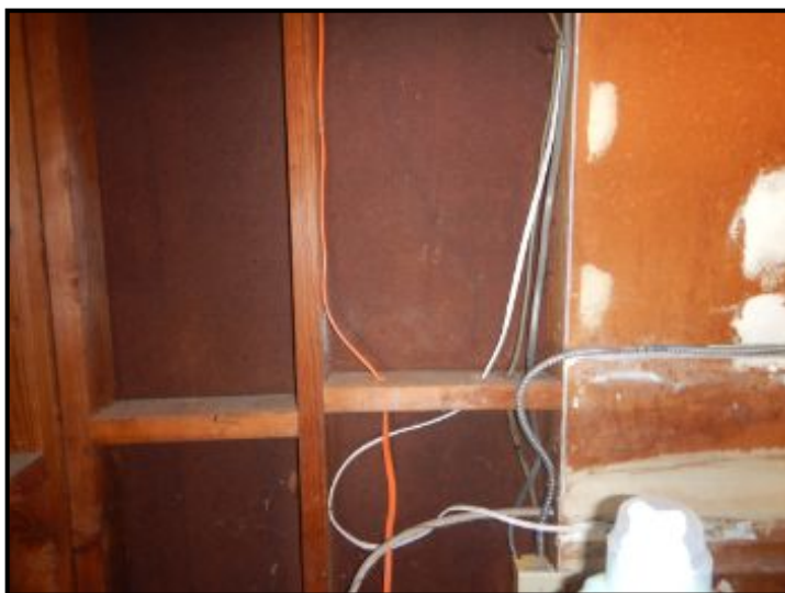
Unprotected romex in garage.
