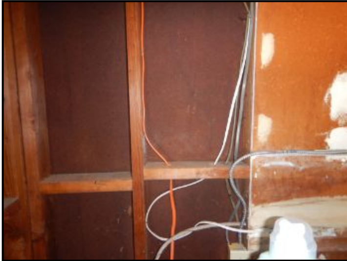
Unprotected romex in garage.
