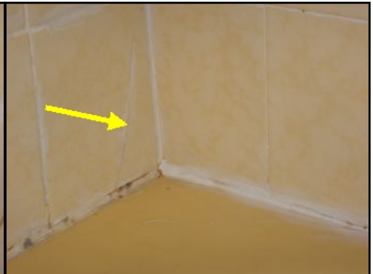
Cracked tiles at bathroom shower.
