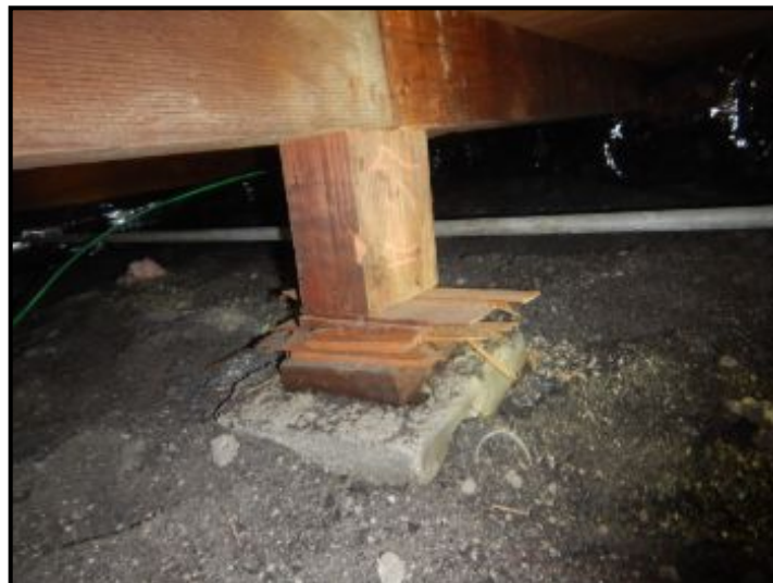
Shims used at concrete piers.
