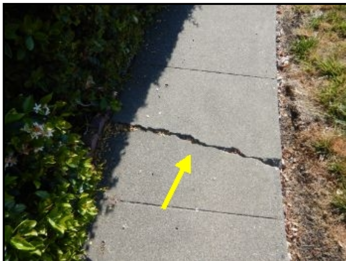
Cracking to walkways.
