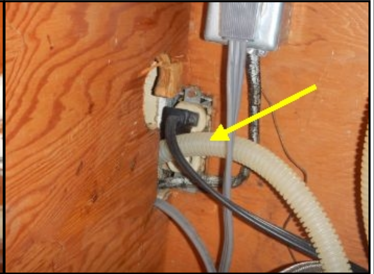
Missing cover plate under the kitchen sink.
