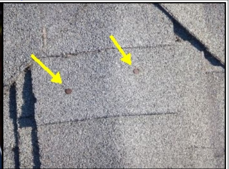
Exposed ridge fasteners.
