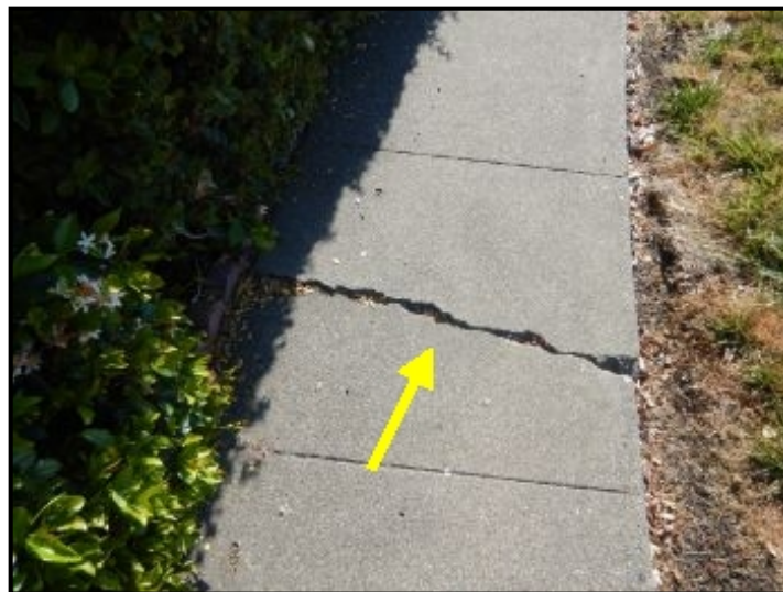
Cracking to walkways.
