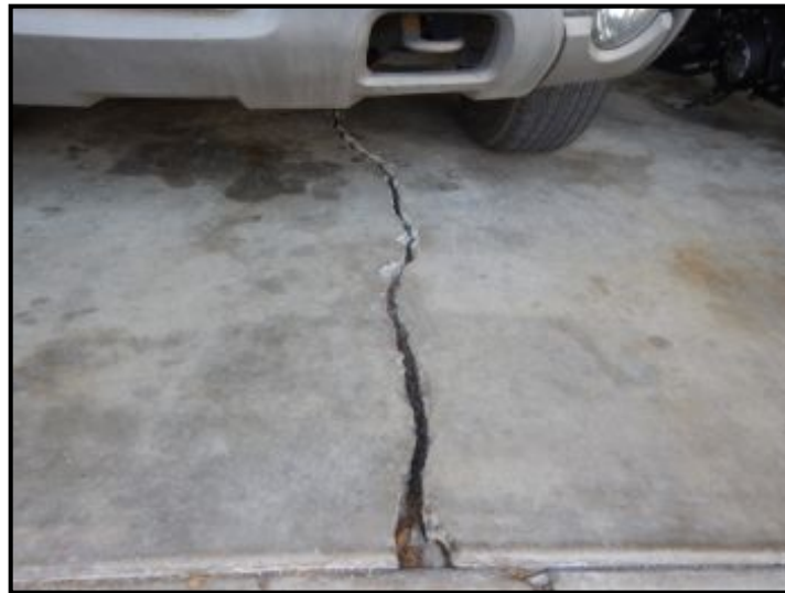
Cracking at garage floor.
