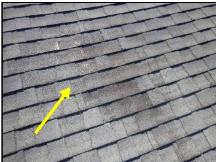
Worn section of roofing shingles.
