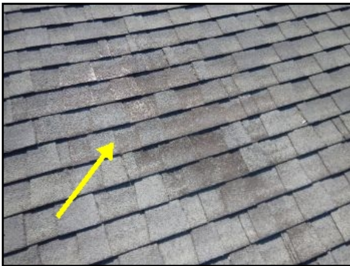
Worn section of roofing shingles.
