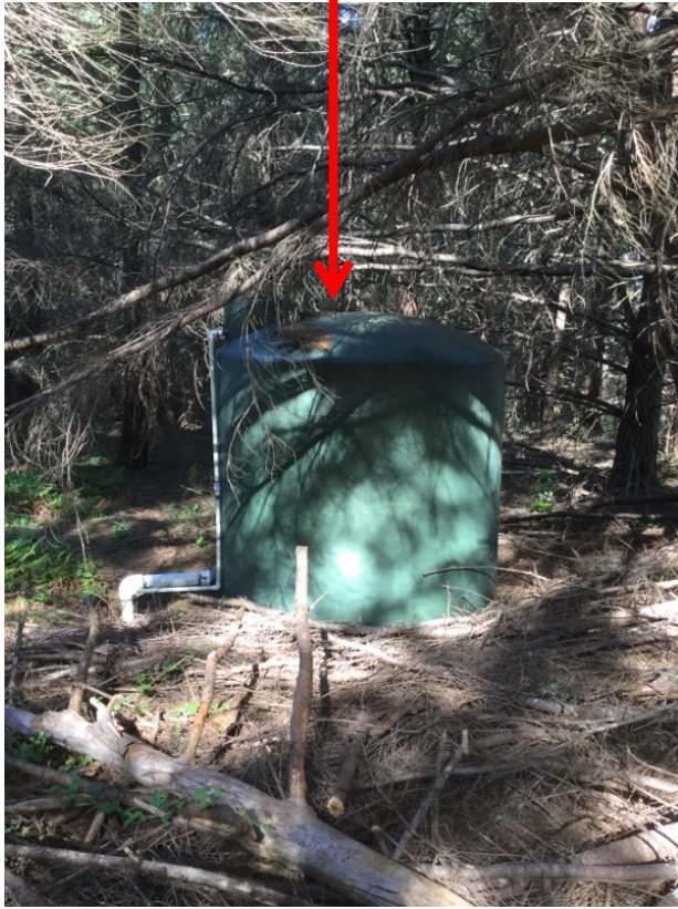
Fire Protection Tank
