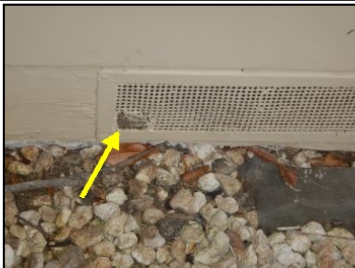
Seal vent screen at rear of garage.
