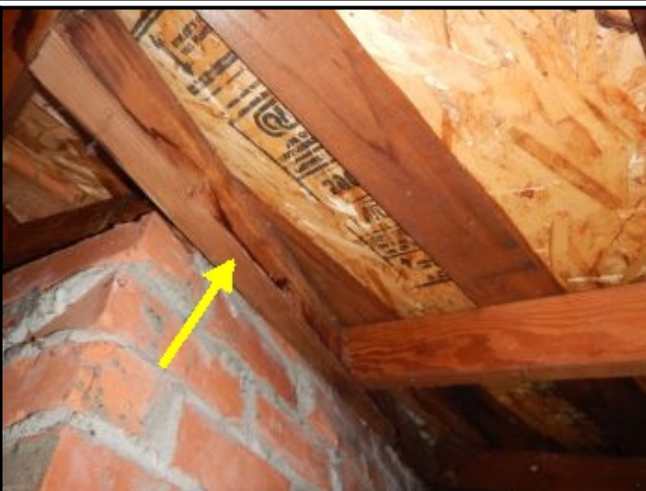
Moisture staining around chimney in attic.
