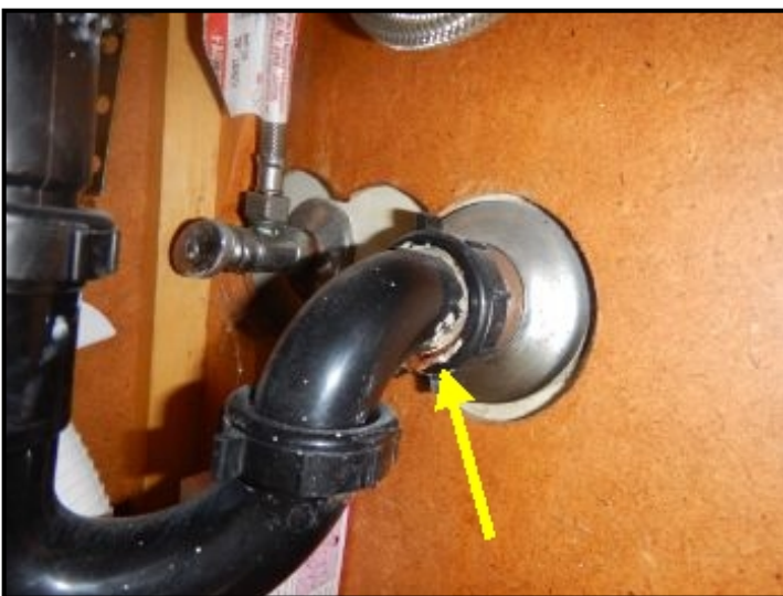
Leaking at half bathorom sink.
