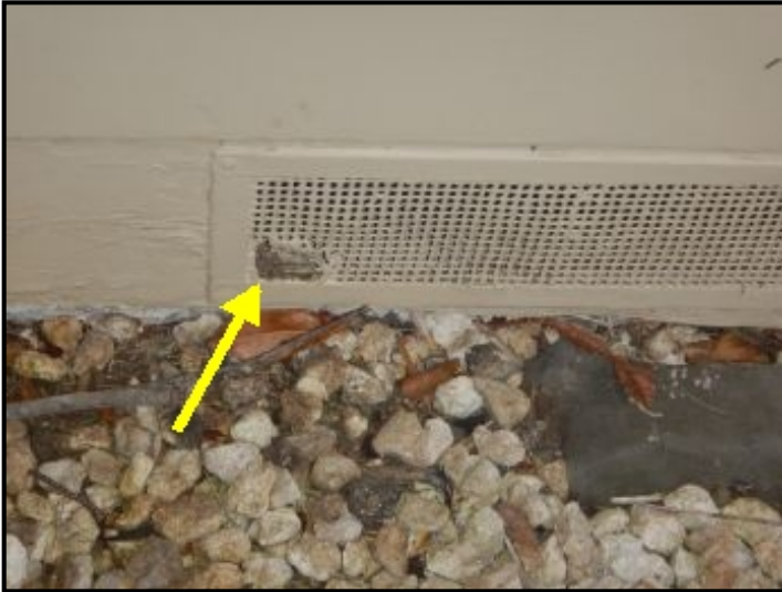
Seal vent screen at rear of garage.
