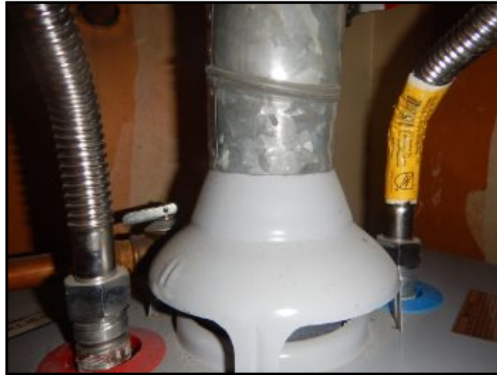
Install screws at flue/flue hood.
