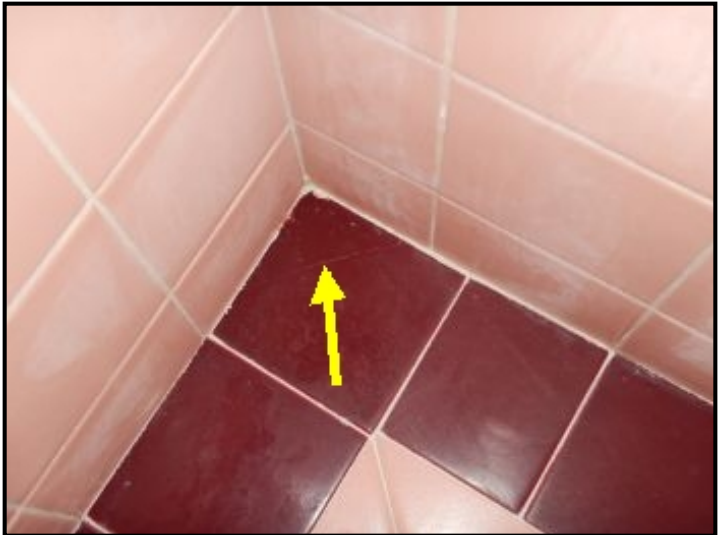
Cracked tile at master bathroom shower.
