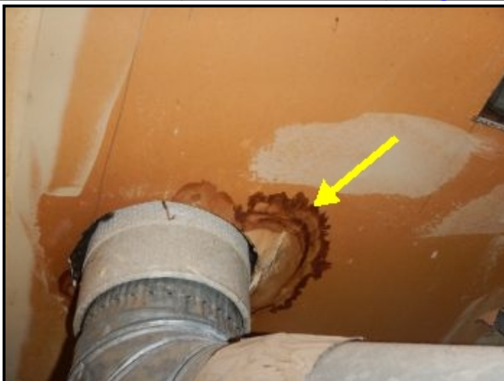
Moisture stains around furnace vent pipe.
