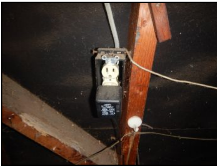
Missing cover plate in garage.
