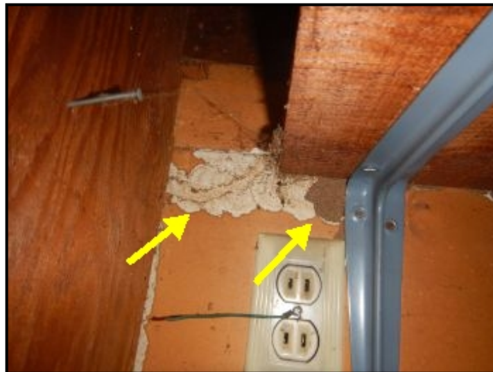
Apparent termite activity in the garage.
