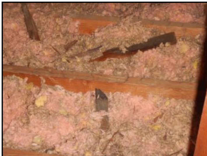
Low insulation in the attic.
