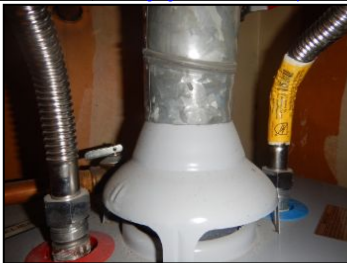
Install screws at flue/flue hood.
