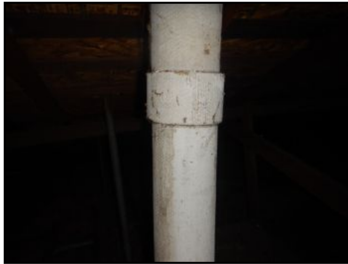
Older transite pipes in attic.
