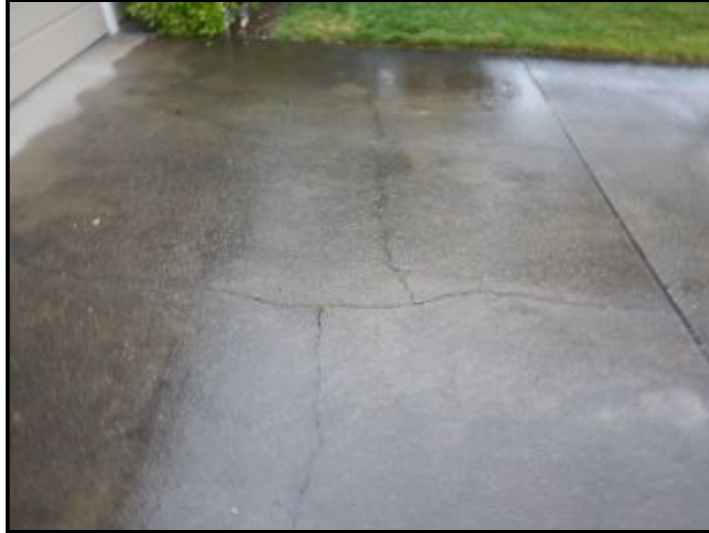
Cracking at driveway.
