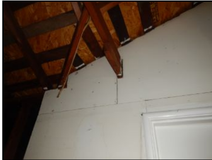
Seal firewall as needed.
