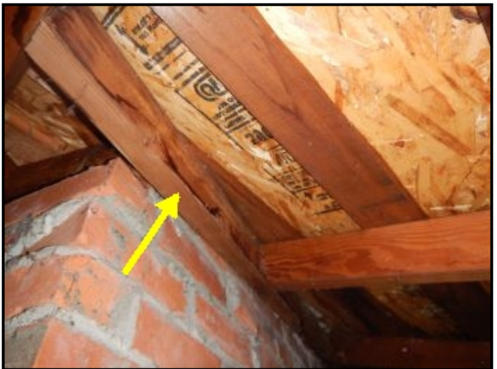
Moisture staining around chimney in attic.
