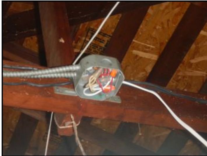
Missing junction box cover in the garage.
