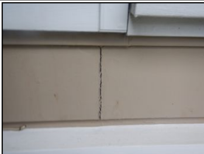
Caulk/seal gaps at siding as needed
