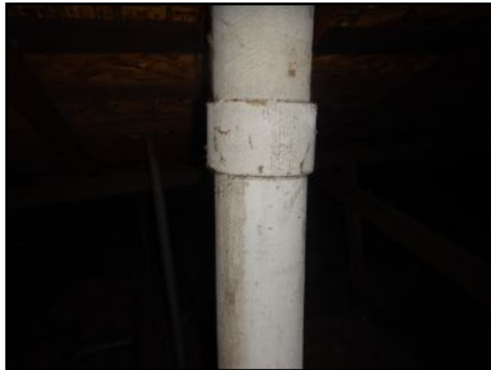
Older transite pipes in attic.
