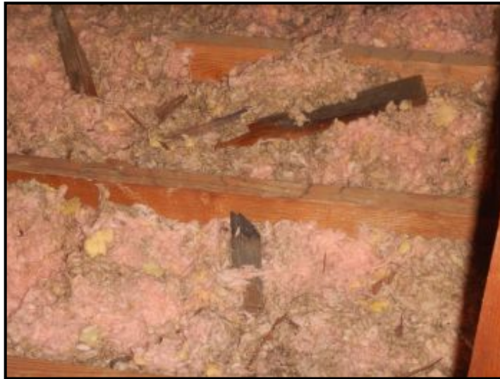
Low insulation in the attic.
