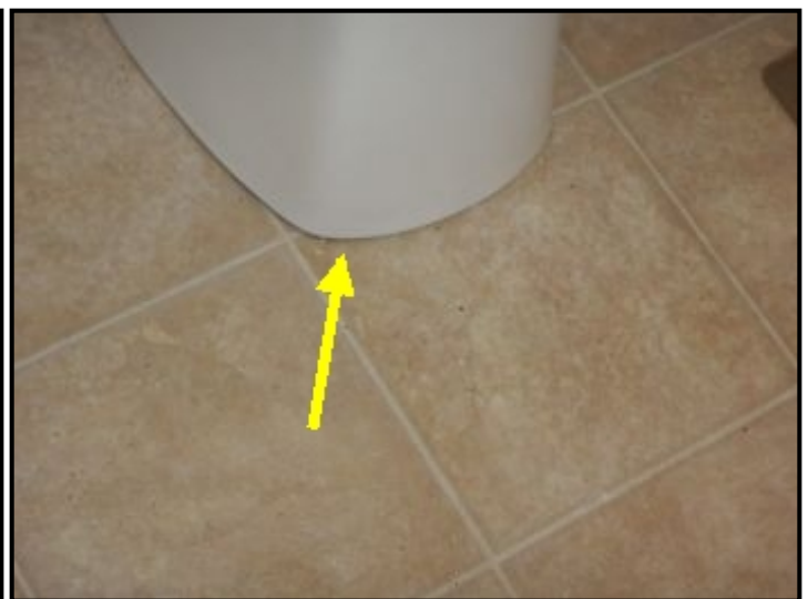
Leaking from toilet seal at half bathroom.
