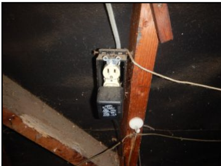
Missing cover plate in garage.
