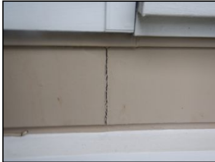
Caulk/seal gaps at siding as needed
