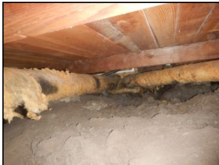
Deteriorated/missing insulation to ducting.
