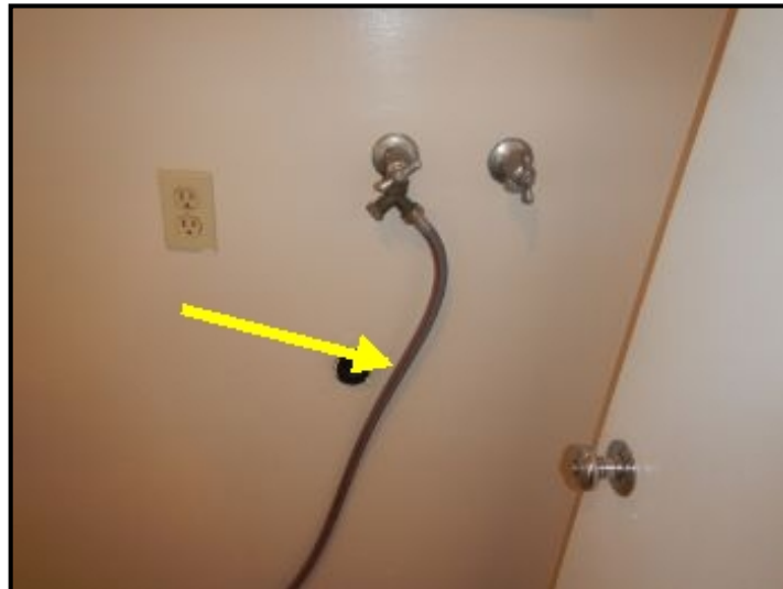
Hose installed from water supply into garage for sink.
