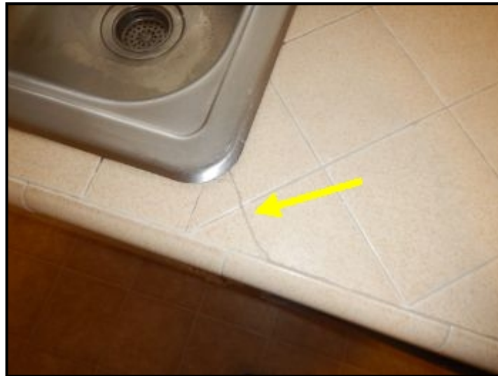
Cracked tiles noted at counter tops.
