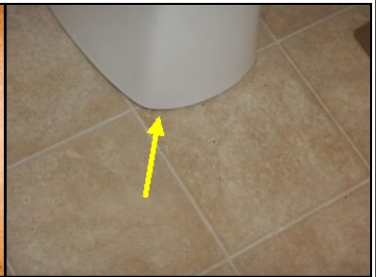
Leaking from toilet seal at half bathroom.
