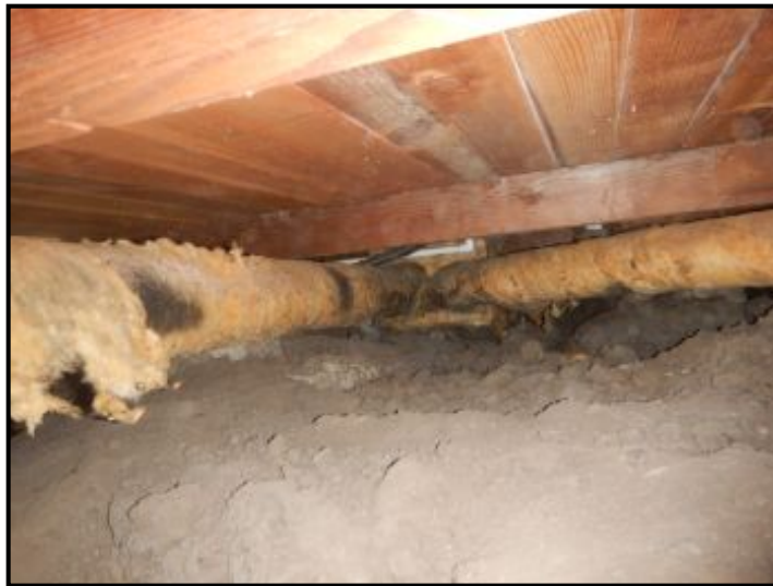
Deteriorated/missing insulation to ducting.
