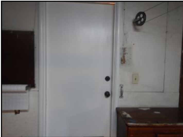
Garage door is not a fire rated door.
