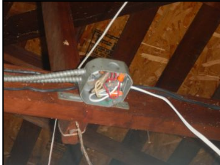
Missing junction box cover in the garage.
