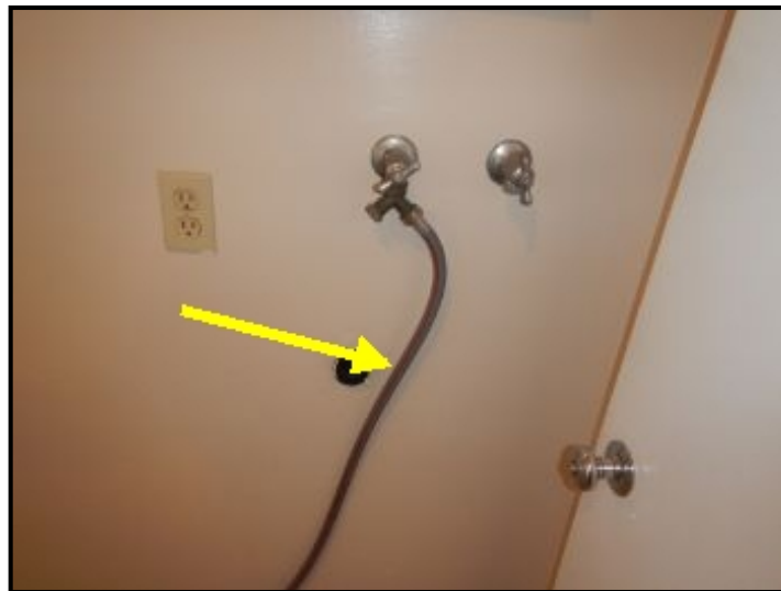
Hose isntalled from water supply into garage for sink.
