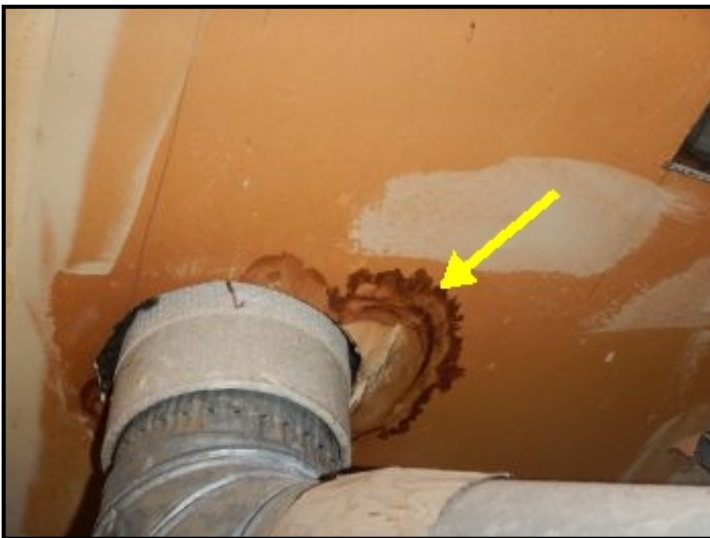
Moisture stains around furnace vent pipe.
