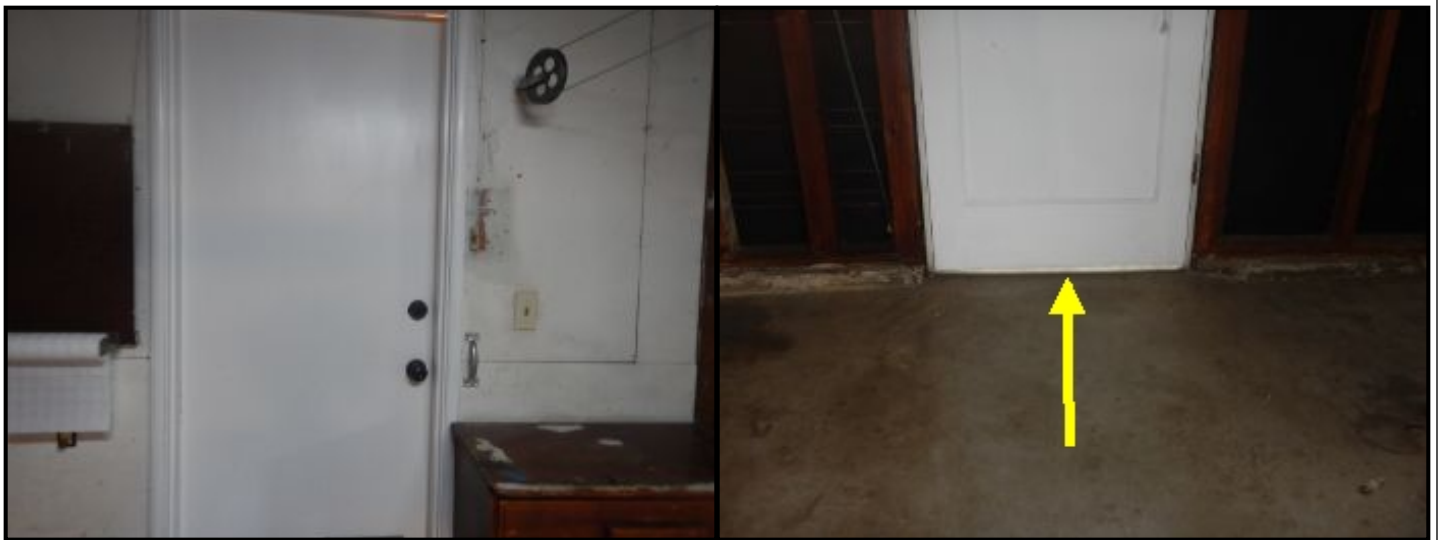
Garage door is not a fire rated door.
