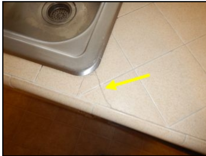
Cracked tiles noted at counter tops.
