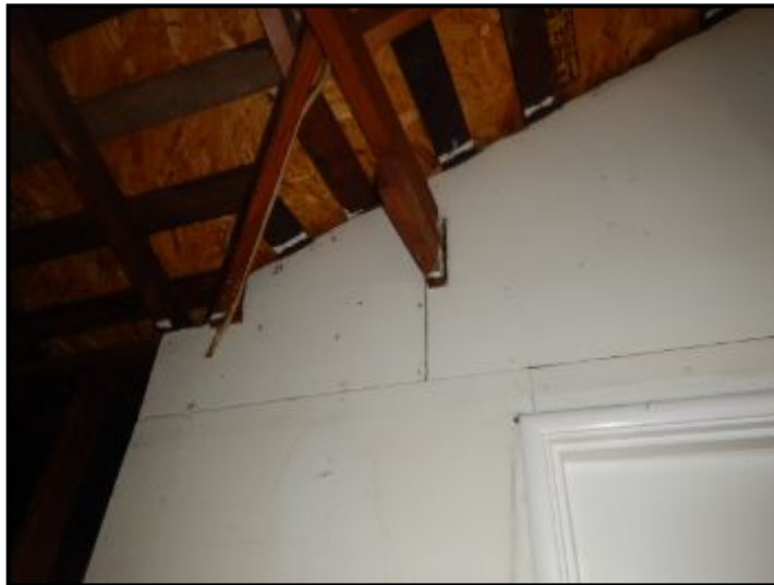
Seal firewall as needed.
