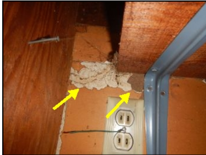
Apparent termite activity in the garage.
