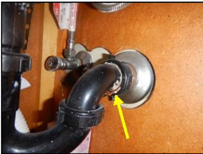
Leaking at half bathorom sink.
