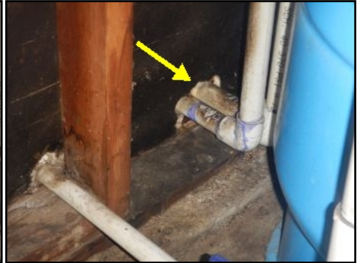
Seal around pipes at back of garage.
