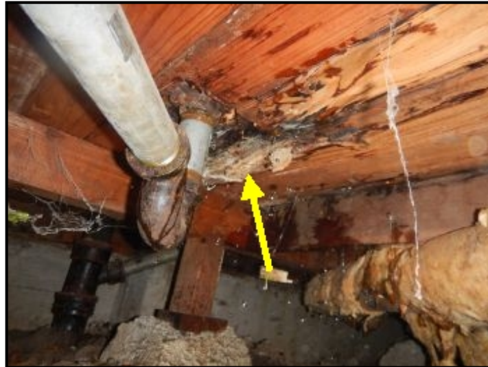
Wood damage to sub floor of master bathroom.
