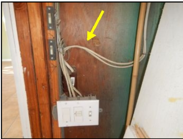
Unprotected electrical at the garage.
