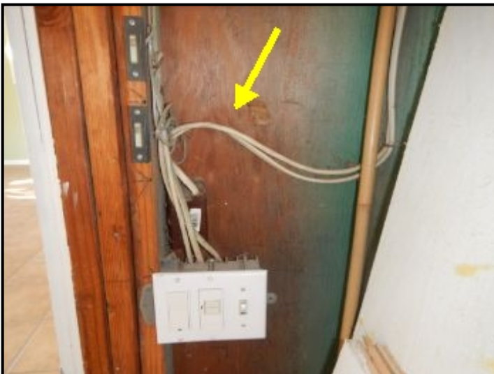
Unprotected electrical at the garage.
