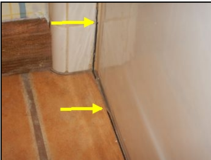
Grout voids at tub/wall in hall bathroom.
