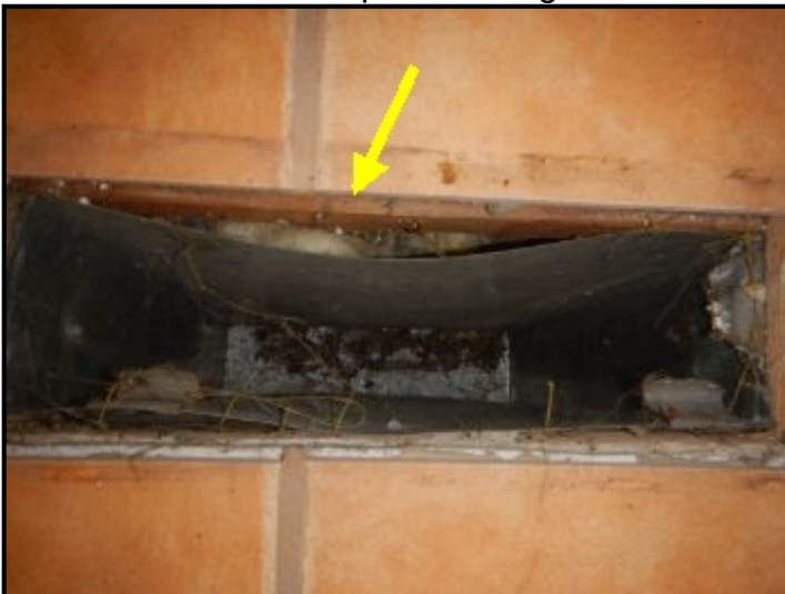
Seal floor heat registers as needed.
