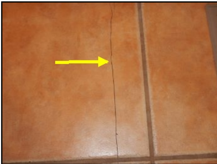
Cracked tiles at bathroom floor.
