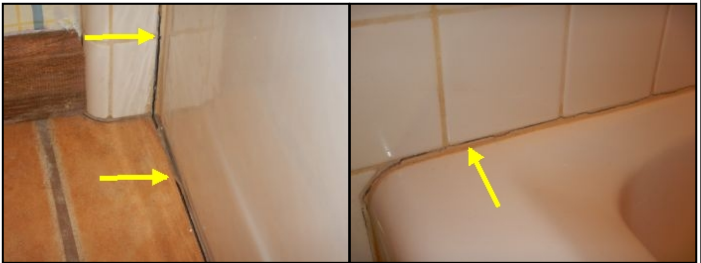
Grout voids at tub/wall in hall bathroom.
