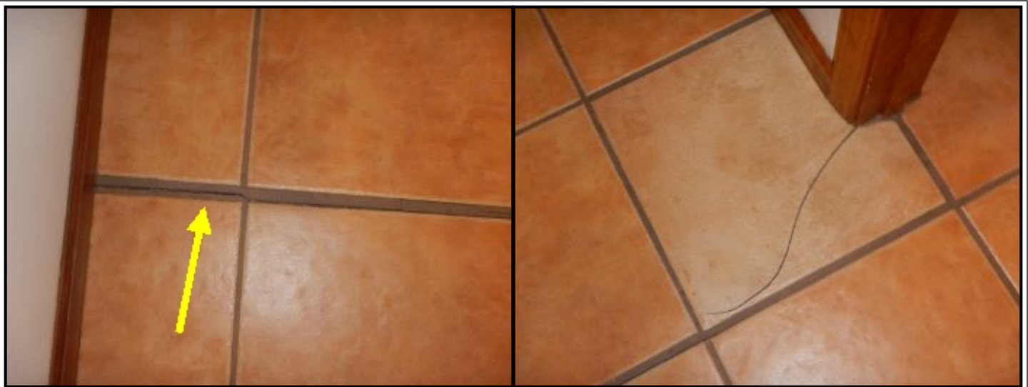
Cracking grout at hallway tile.
