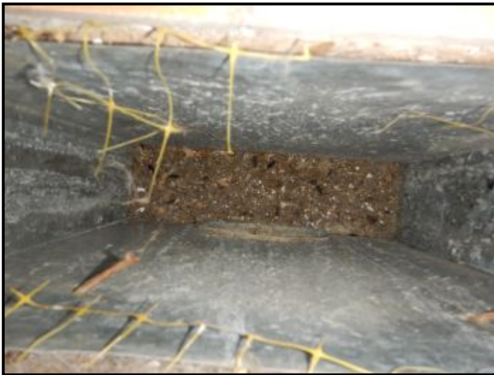
Debris build up in heat registers.
