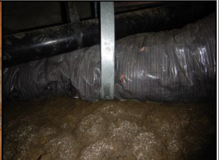
Heating duct sitting on the ground in the sub area.
