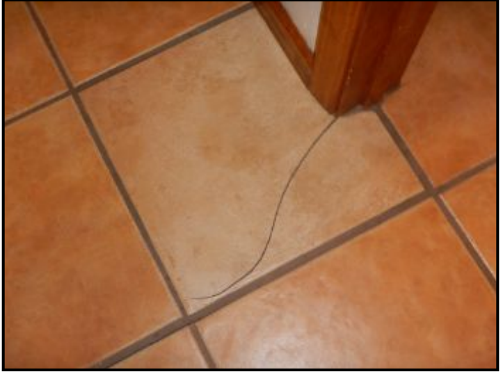
Cracked tile at hallway.
