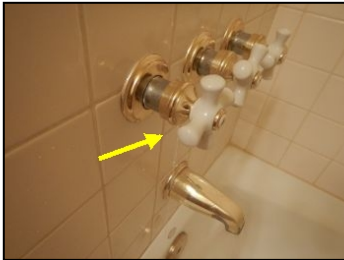
Leaking shower fixture at hall bathroom.
