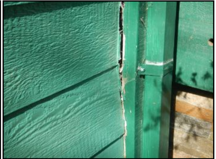
Bulging siding at right side of home.
