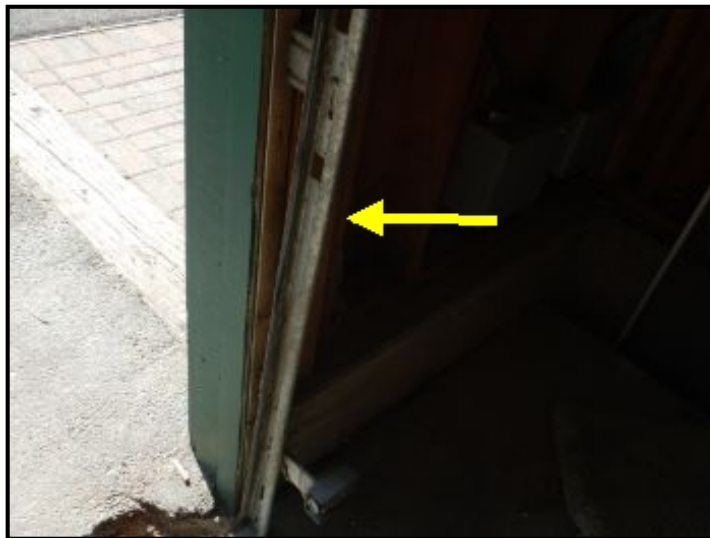
Bent/warped track at garage door.
