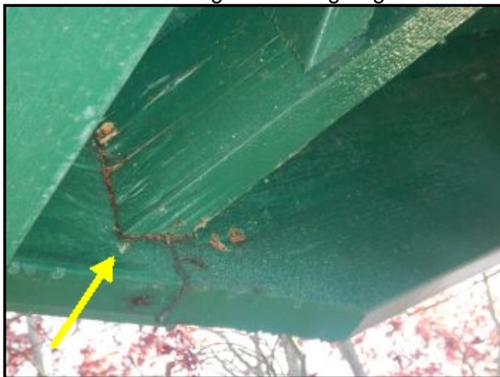
Fascia damage at right side of home.
