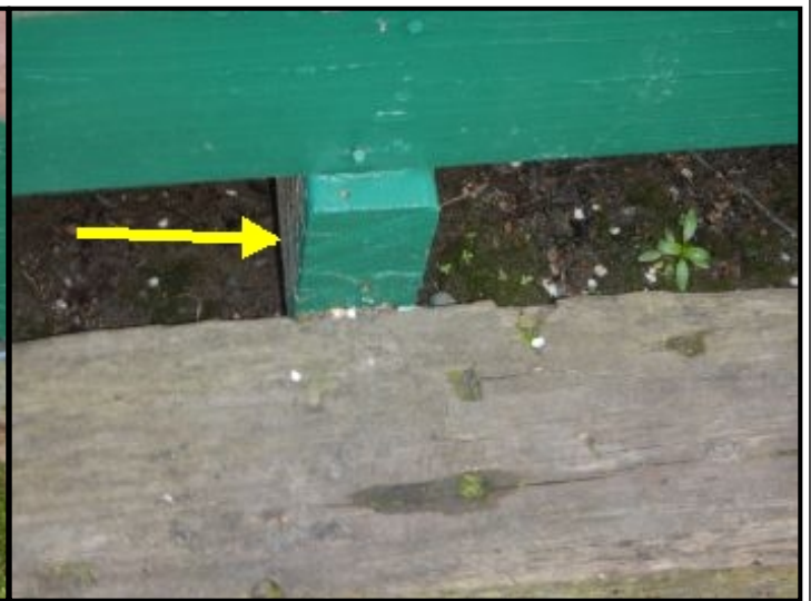
Damage to ends of girders at rear deck.
