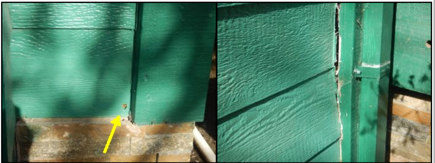
Siding damage to right of garage door.
