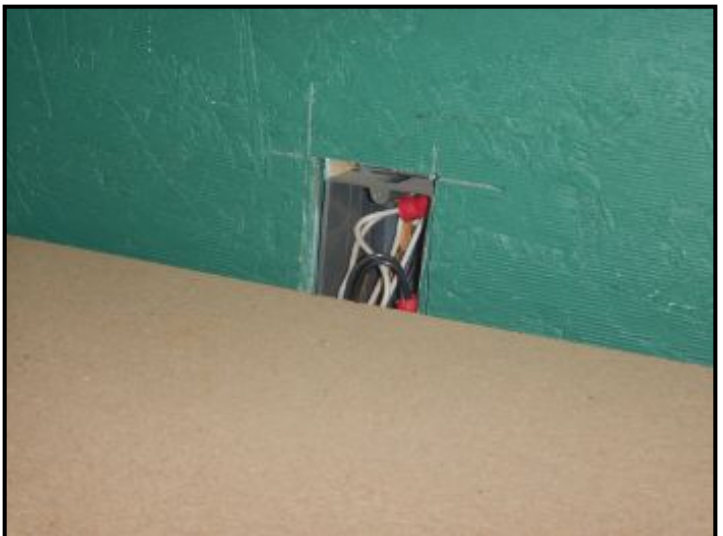
Missing junction box cover in garage cabinet.
