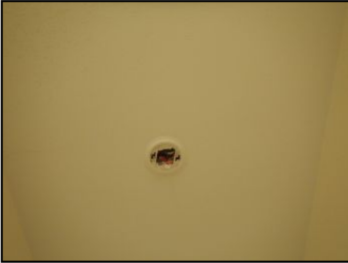
Missing smoke detector at hallway.
