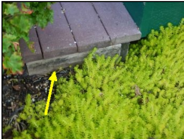
Earth/wood contact at rear deck steps.
