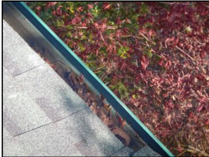
Standing water/debris in right side gutter.
