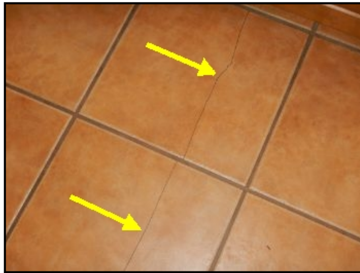
Cracking tiles at kitchen floor.
