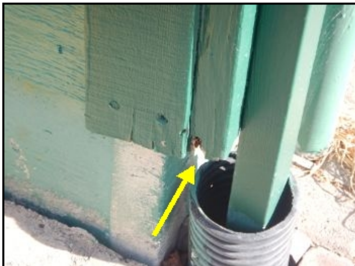
Trim damage at left of garage.
