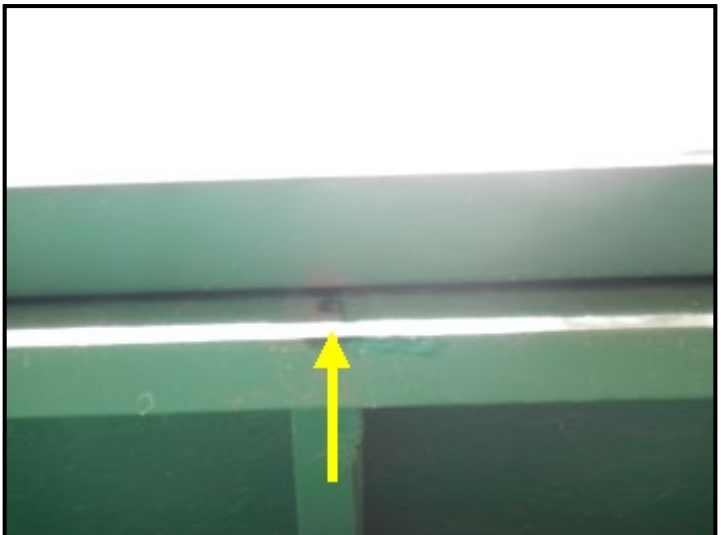
Leaking gutter over garage.
