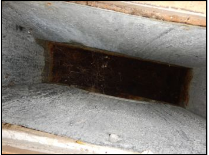
Rust/corrosion to heat register in dining room.
