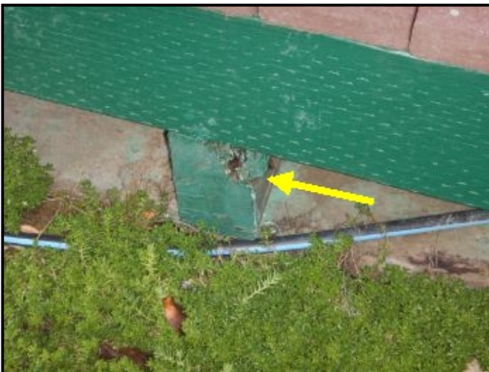
Damage to ends of girders at rear decks.
