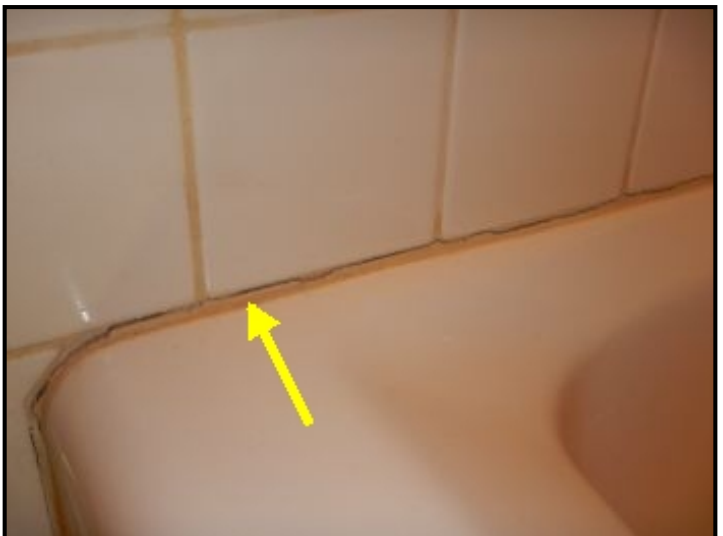
Grout voids around tub at hallway bathroom.
