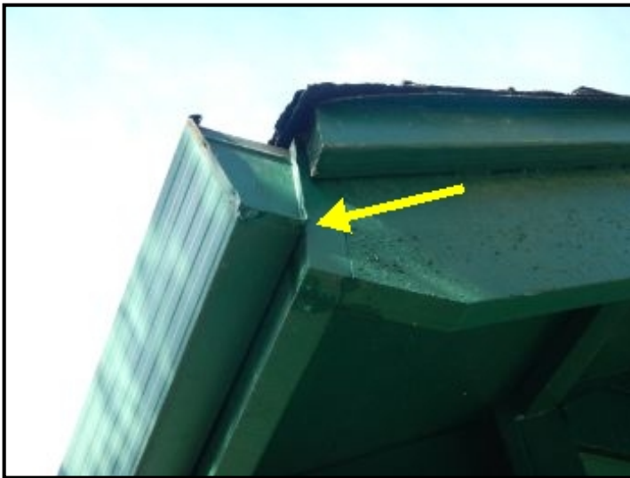
Leaking gutter over garage.
