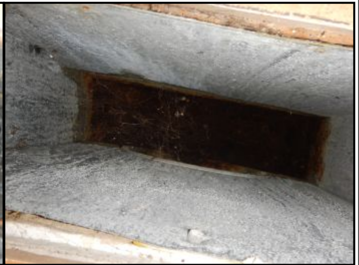
Rust/corrosion to heat register in dining room.
