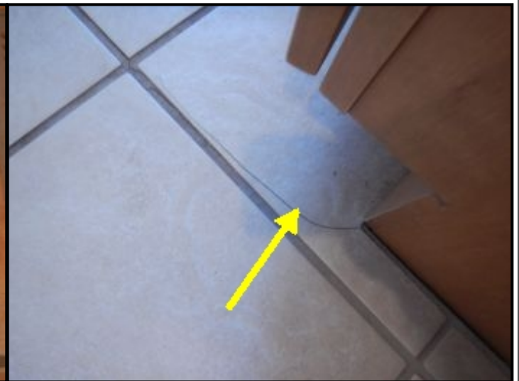
Cracked tiles at master bathroom.
