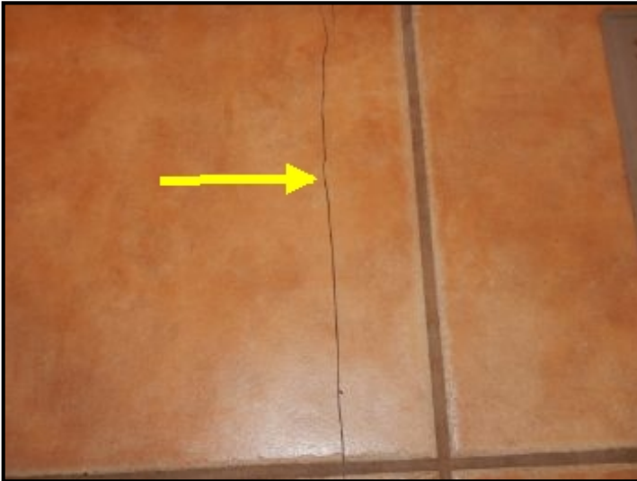
Cracked tiles at bathroom floor.
