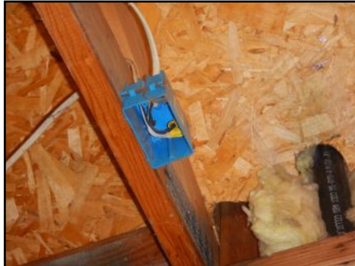
Missing junction box cover in garage.
