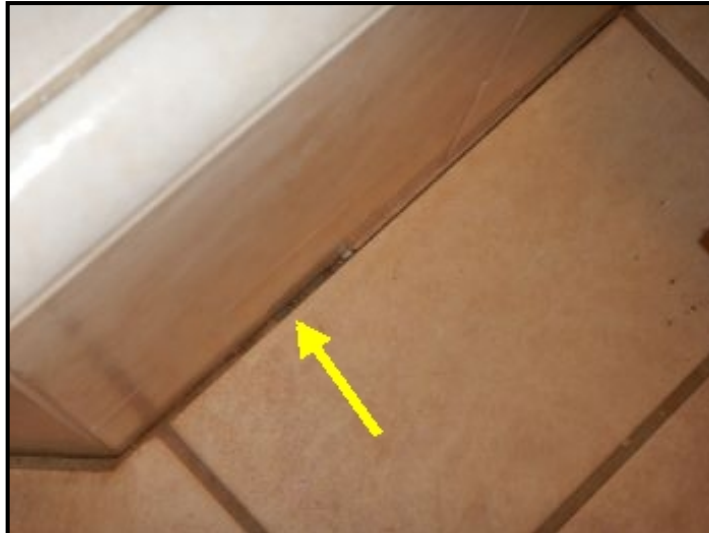
Grout voids at base of master bathroom tub.
