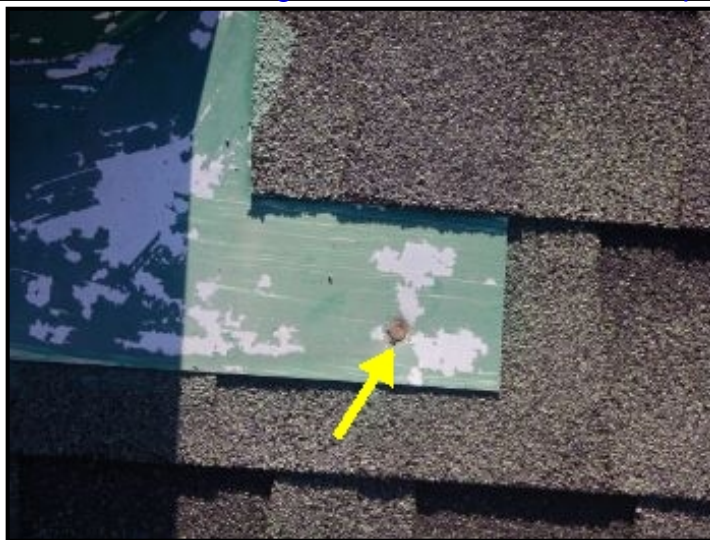
Seal exposed fasteners at roof top flashings.
