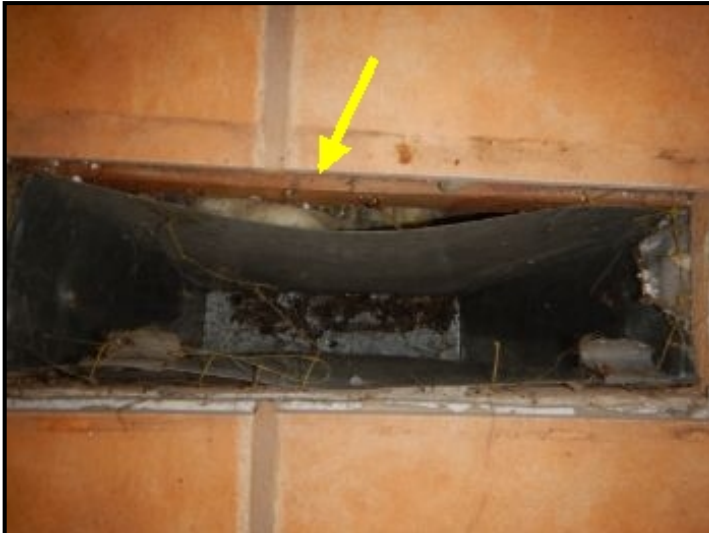
Seal floor heat registers as needed.
