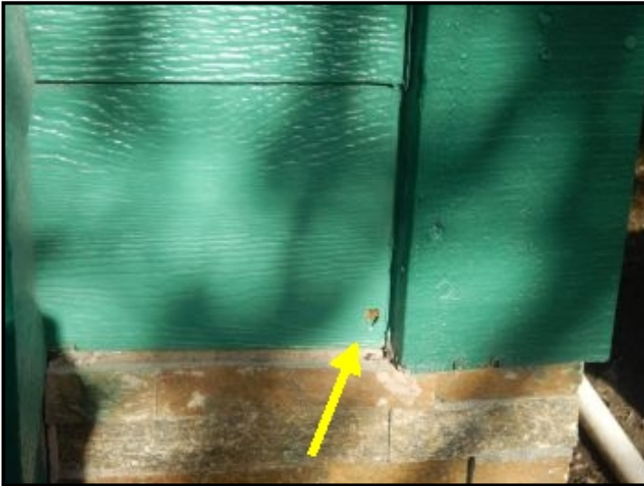
Siding damage to right of garage door.
