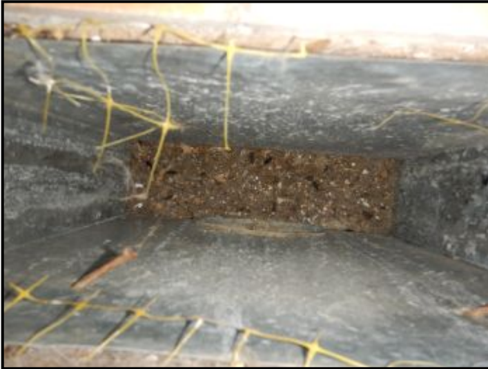
Debris build up in heat registers.
