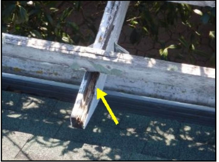
Deterioration of front trellis.
