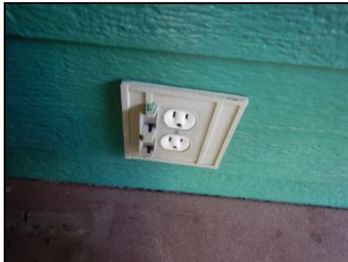
Replace weather protective cover at rear deck.
