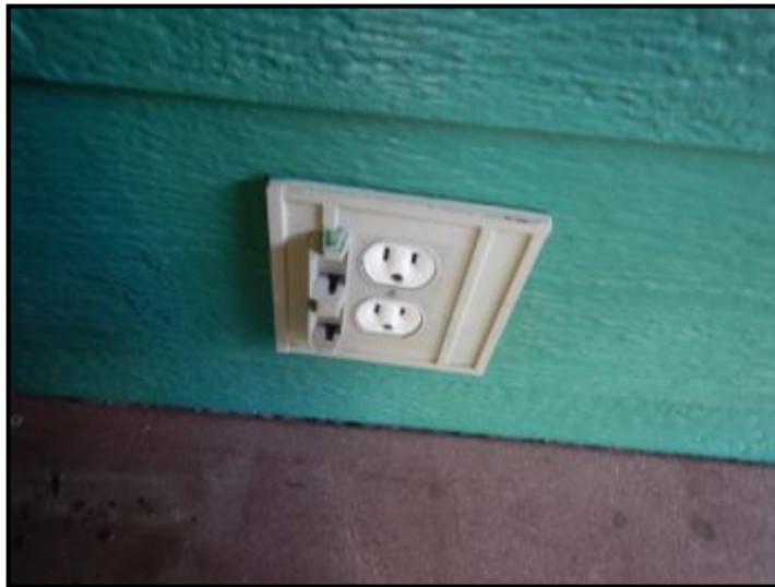
Replace weather protective cover at rear deck.
