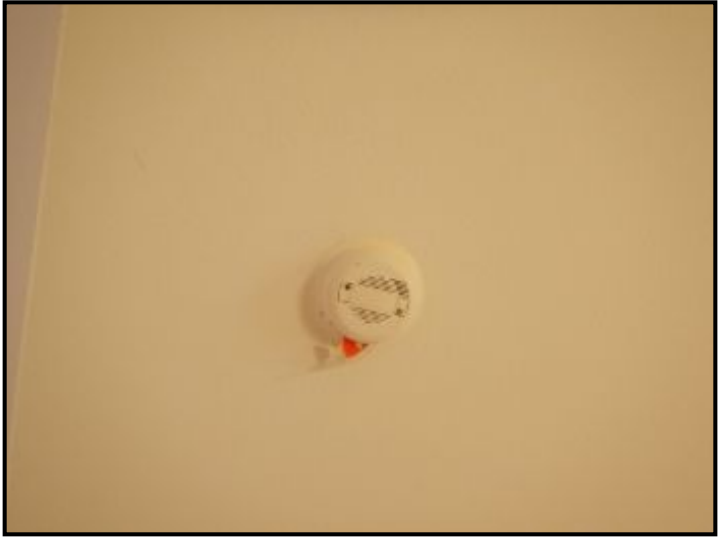
Missing battery at smoke detector.
