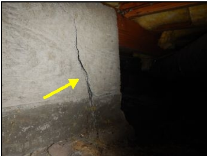
Excessive cracking at foundation wall.
