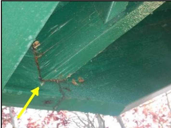
Fascia damage at right side of home.
