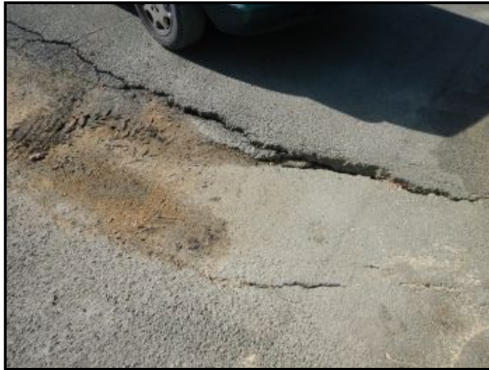
Cracking/settling to driveway.
