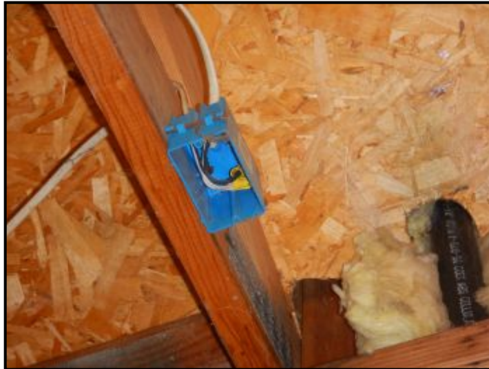
Missing junction box cover in garage.
