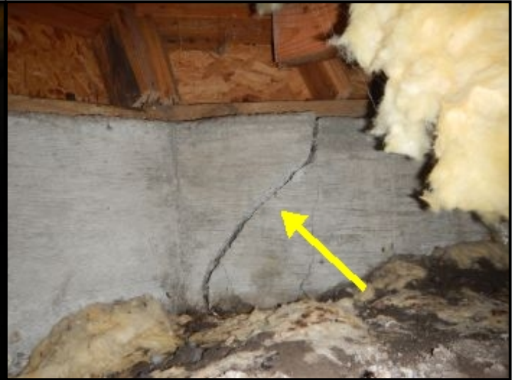
Excessive cracking at foundation wall.
