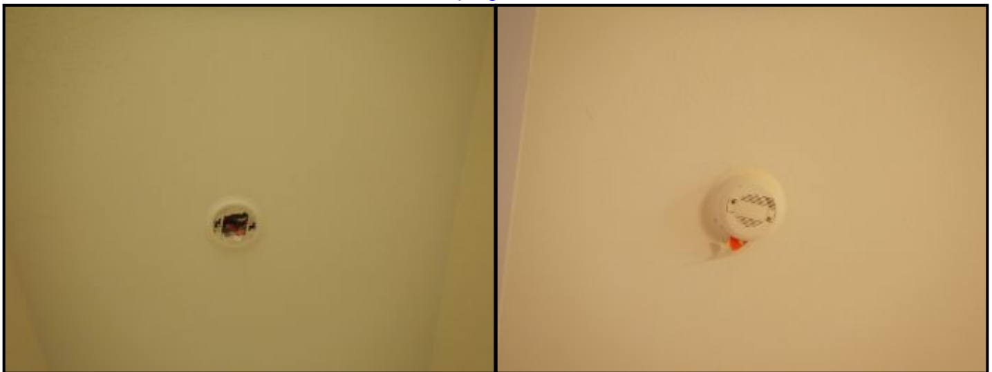
Missing smoke detector at hallway.
