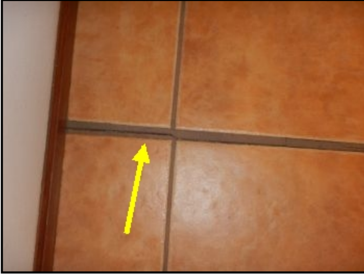
Cracking grout at hallway tile.
