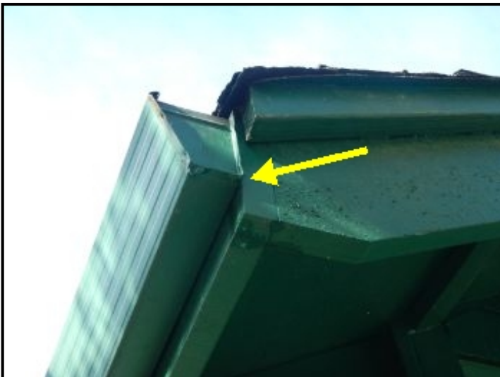
Leaking gutter over garage.
