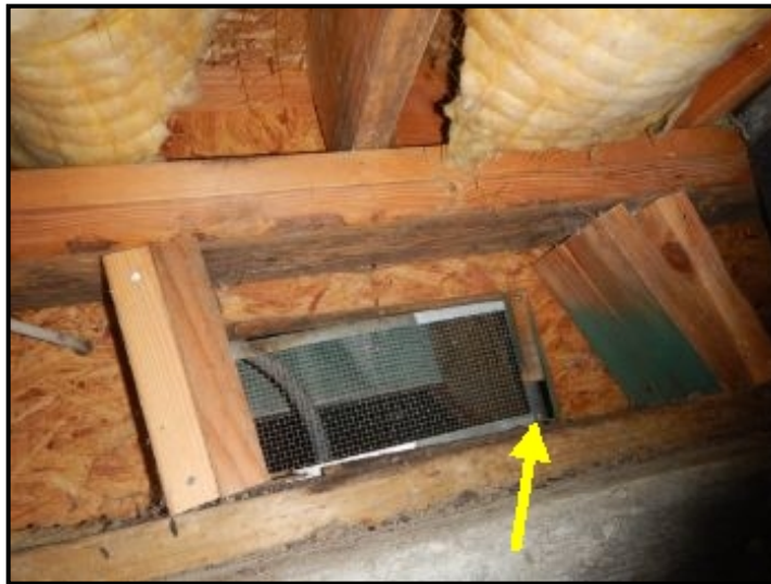
Gaps around vent screens under rear decks.
