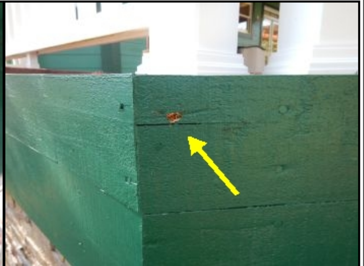
Fascia damage to areas at rear decks.
