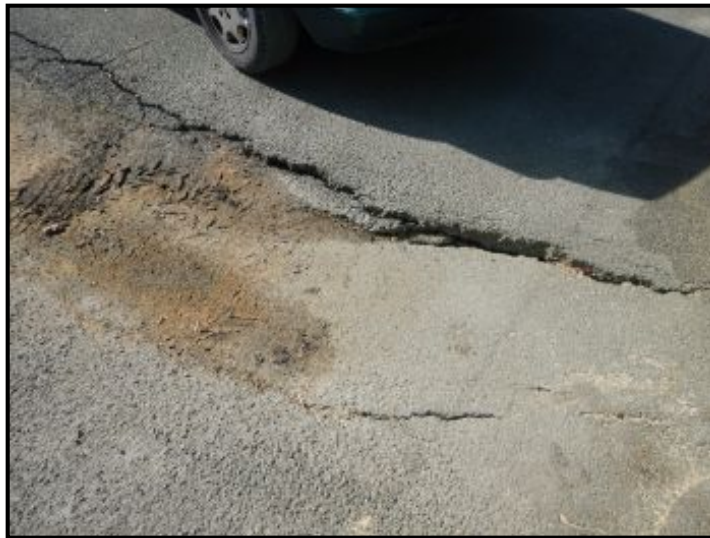
Cracking/settling to driveway.
