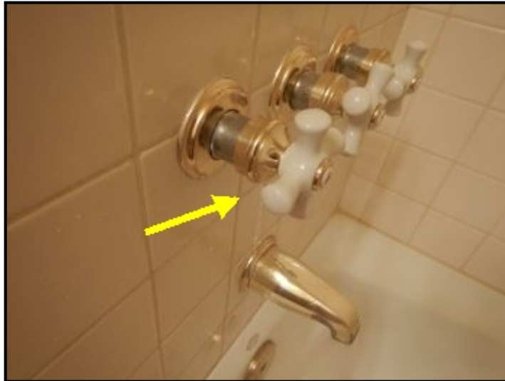
Leaking shower fixture at hall bathroom.
