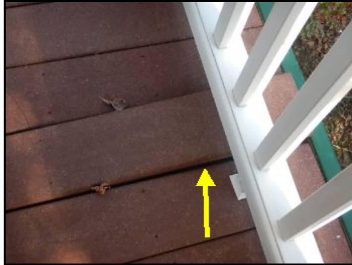
Lifted deck surface board,
