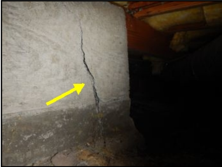
Excessive cracking at foundation wall.
