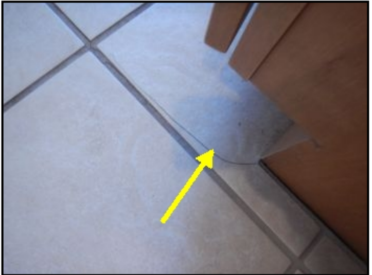
Cracked tiles at master bathroom.
