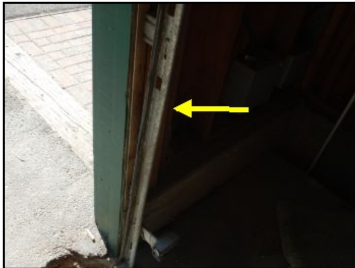
Bent/warped track at garage door.
