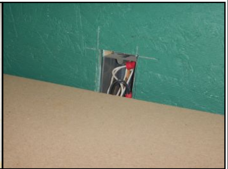
Missing junction box cover in garage cabinet.
