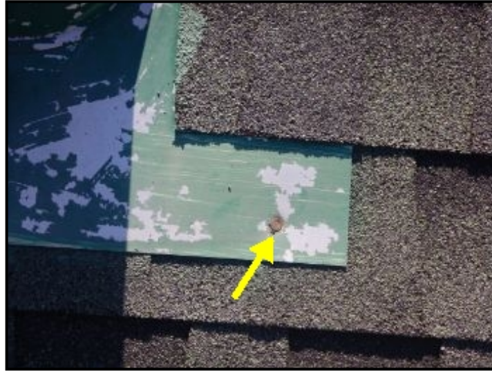
Seal exposed fasteners at roof top flashings.
