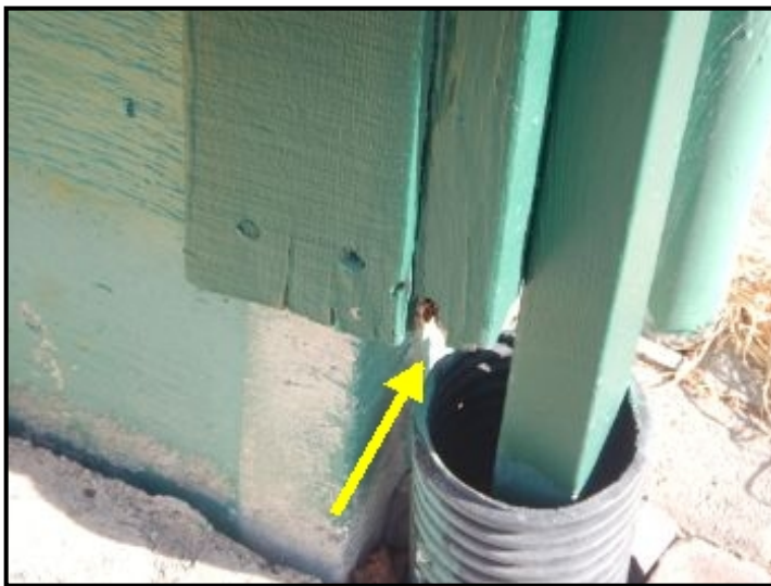
Trim damage at left of garage.
