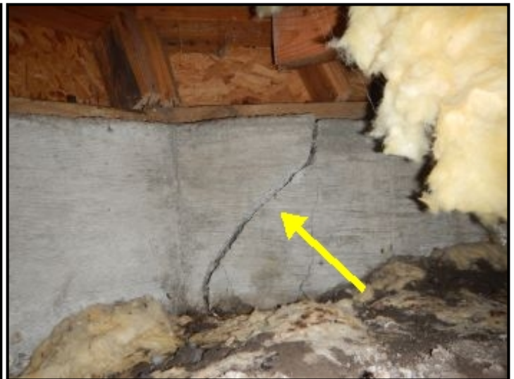
Excessive cracking at foundation wall.
