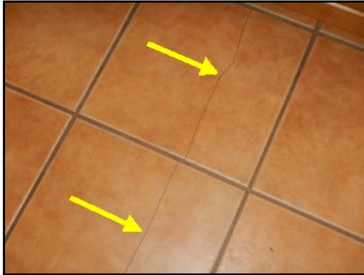
Cracking tiles at kitchen floor.
