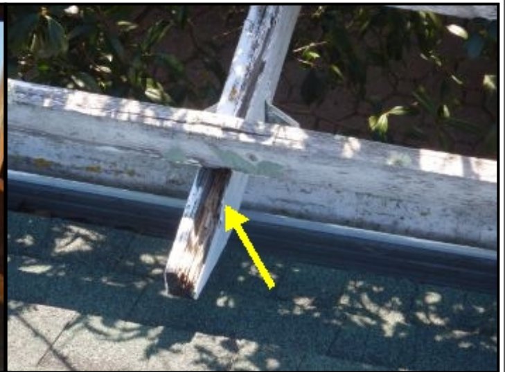
Deterioration of front trellis.
