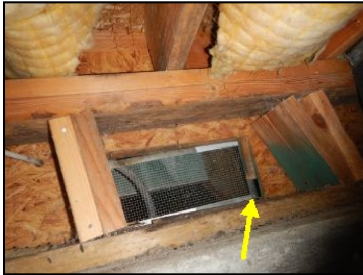
Gaps around vent screens under rear decks.
